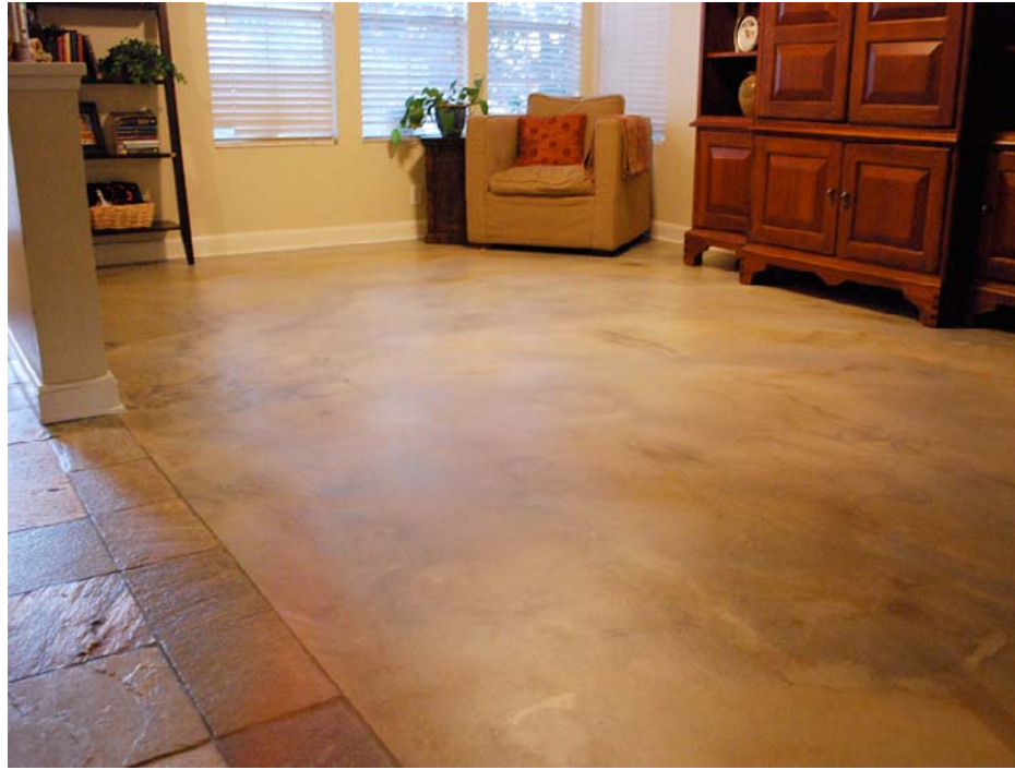
Darius Gross of San Diego-based Life Deck Coating Installations pours Westcoat Specialty Coating Systems' TC-25 on a living-room floor. The material was used to level the room and was poured between 1/4 inch and 1/2 inch thick. It was hard enough to walk on and stain within a few hours. The floor was stained with Westcoat SC-35 Water-Based Stain and Sealed with EC-11 Water-Based Epoxy and EC-96 Satin Polyurethane Topcoat.
