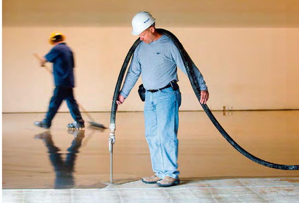
USG Corp.'s Levelrock Proflow is pumped onto a concrete substrate.
