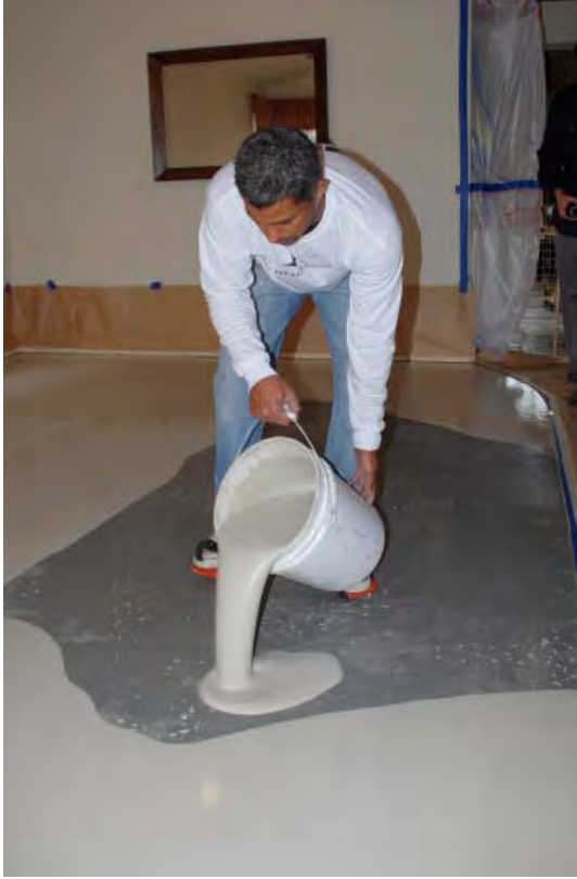
Darius Gross of San Diego-based Life Deck Coating Installations pours Westcoat Specialty Coating Systems' TC-25 on a living-room floor. The material was used to level the room and was poured between 1/4 inch and 1/2 inch thick. It was hard enough to walk on and stain within a few hours. The floor was stained with Westcoat SC-35 Water-Based Stain and Sealed with EC-11 Water-Based Epoxy and EC-96 Satin Polyurethane Topcoat.
