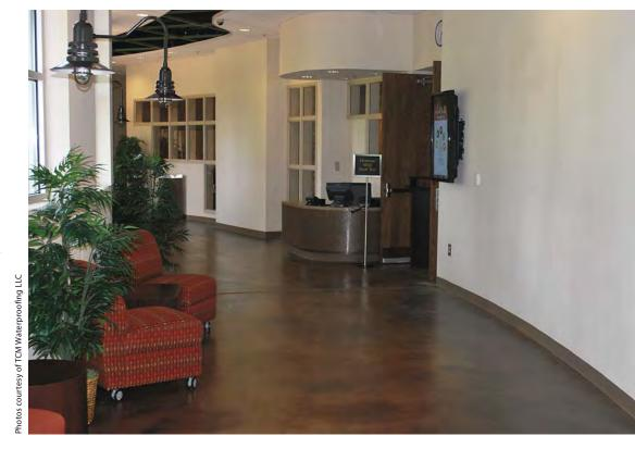
garage. "You don't want to close the floor too much because if you do, you won't get color penetration," he explains. He suggests leaving the floor rough, applying the colorant twice, then running over the floor with a burnisher and a hogshair burnishing pad. The process produces a matte sheen.
