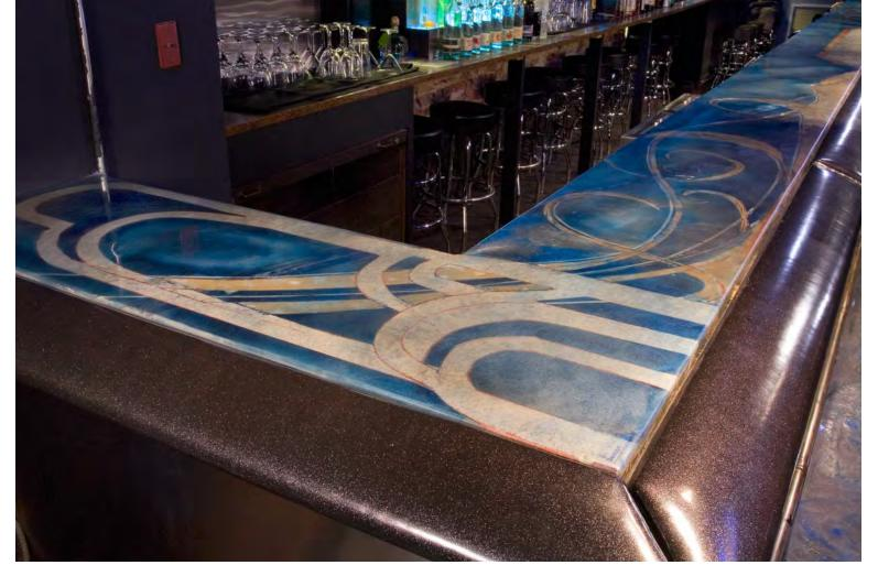
Chocolate and Walnut. Finally, Ryan filled in the engraved lines with Elite Crete's E100-PT1 Fast Clear Epoxy mixed with Elite Crete's Reflector Enhancer, an Elite Crete admixture that produces shimmer and texture, in Brass to make the epoxy nontransparent. He finished the entire floor with a topcoat of the same epoxy mixed with a hint of the Brass Reflector Enhancer. The front lobby was completed in three days.
