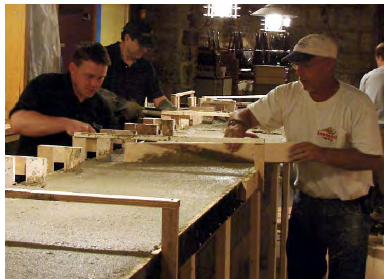
Placing the concrete quickly is key. We had both bars cast in about an hour.
