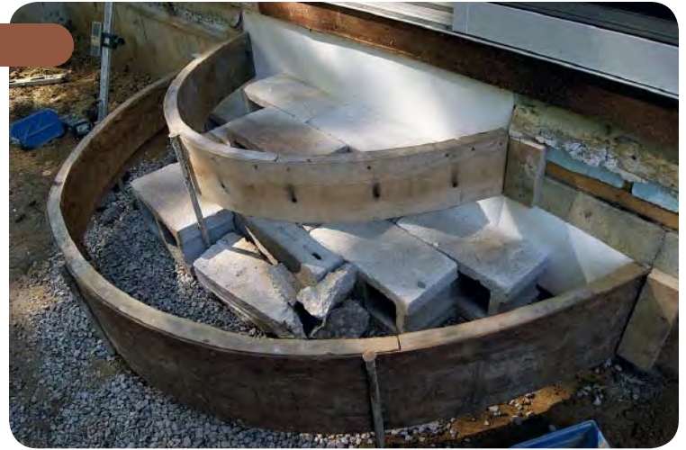
To make sure your forms don't move, fasten blocks of wood to the house at the level the risers will be at. Then, fasten the ends of the forms to the blocks.
