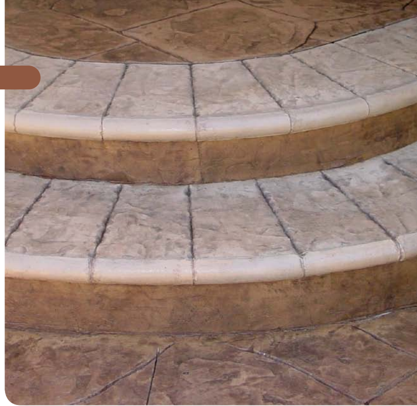
Steps are one of the most visible elements of a project. To make sure you give them your full attention, plan to pour them separately from the rest of your job.
