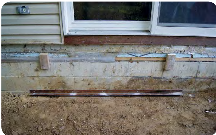
Attach a piece of angle iron to anchor your steps and keep them from sinking.
