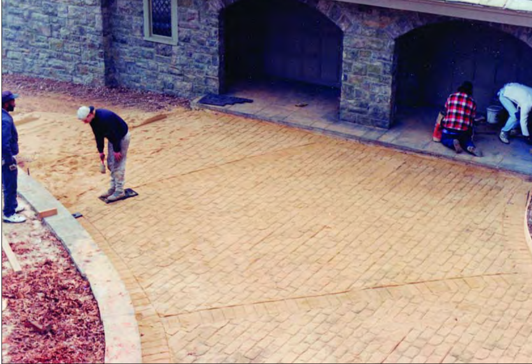
Left: Stamping sand so that the customer can visualize what the drive will look like. This also gives inexperienced workers practice.
