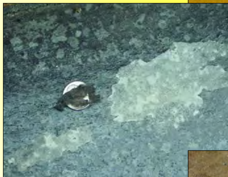
Stain residue creating sealer delaminating issues.
