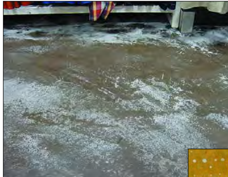
Trapped moisture under the sealer.
