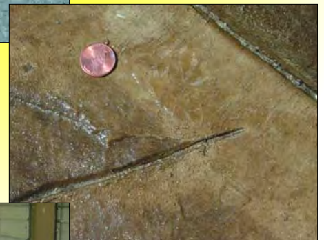
Cracking of sealer film created by over-application.
