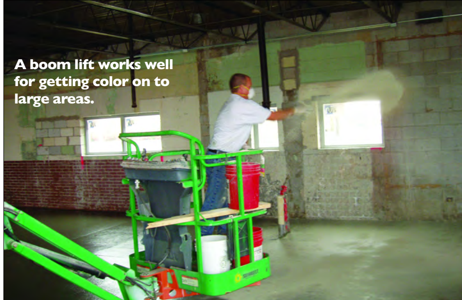
Technique is important. Try and throw the material from knee level or lower so the material does not segregate.
