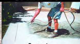
Cement Sprayed On Like Paint
