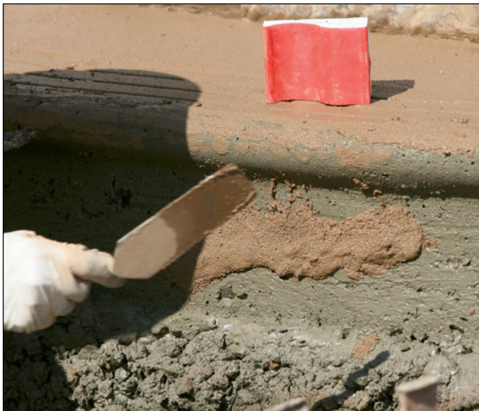
Coloring the face of the step.
