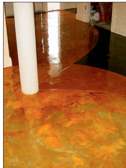
Dave Pettigrew of Diamond D Co. used decorative overlays to give new life to the Prophet Elias Greek Orthodox Church in Santa Cruz, Calif. The original floor consisted of linoleum over plywood. Pettigrew put down a 1/2-inch thick overlay, which was then sawcut and stained with five colors.
