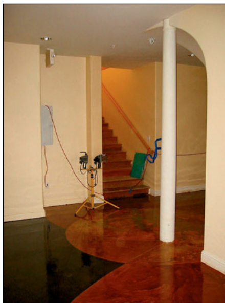
Dave Pettigrew of Diamond D Co. used decorative overlays to give new life to the Prophet Elias Greek Orthodox Church in Santa Cruz, Calif. The original floor consisted of linoleum over plywood. Pettigrew put down a 1/2-inch thick overlay, which was then sawcut and stained with five colors.
