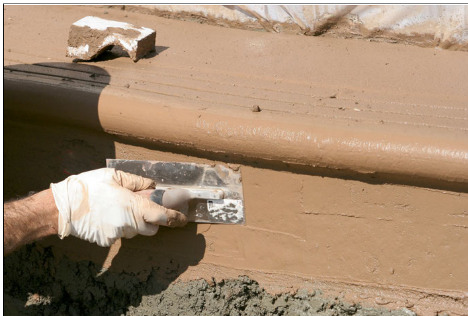
Finishing the step face.
