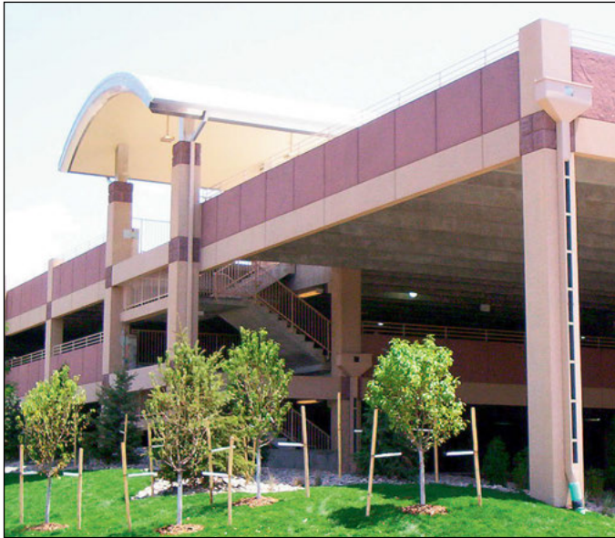
The open system of the Panorama IV parking structure in Denver includes beautifully decorated architectural concrete columns and spandrels on the exterior. The textures were created with form liners.
