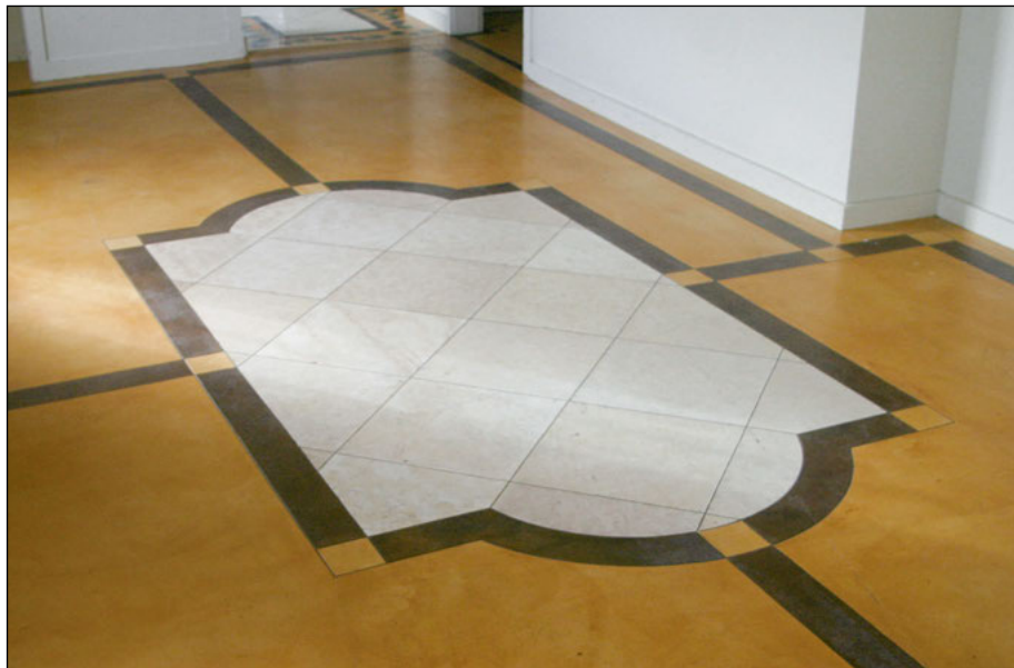
This overlay on a wood subfloor was created with Ardex Products, then colored with acid stains and dyes.
