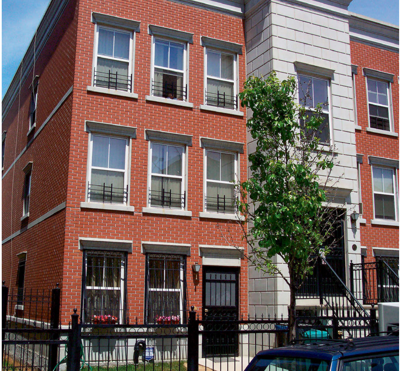
The Melrose Housing Project in the South Bronx was built using Scott System's Brick Snaps for the walls and a traditional form liner for the contrasting entry.
