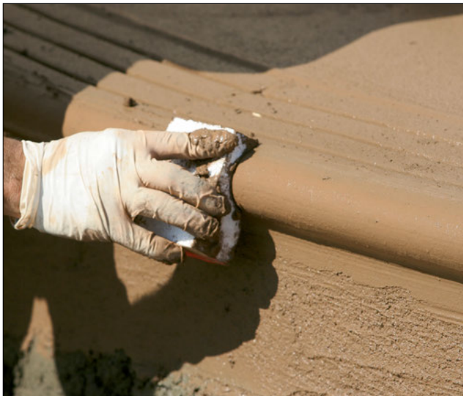
Finishing the bull nose with a profile tool.
