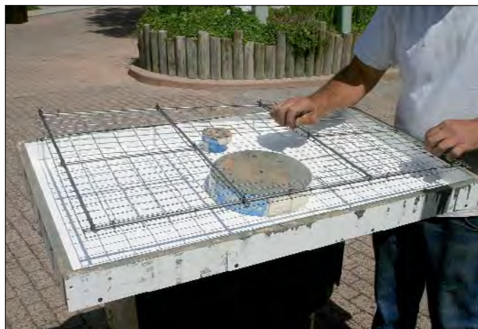
Galvanized wire used for reinforcement in a backsplash.
