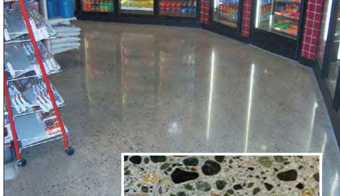
RetroPlate with exposed aggregate in a retail setting.
