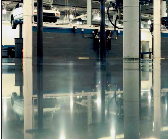
Flat floor with polished cream, no fines or aggregate.
