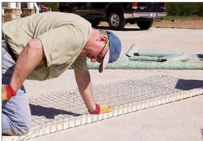
C-Grid is used around a sink hole.
