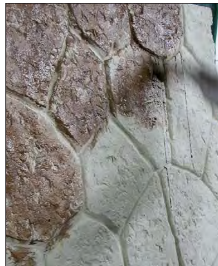
Maurizio Pontello demonstrates Ideal Work's vertical overlayment system.
