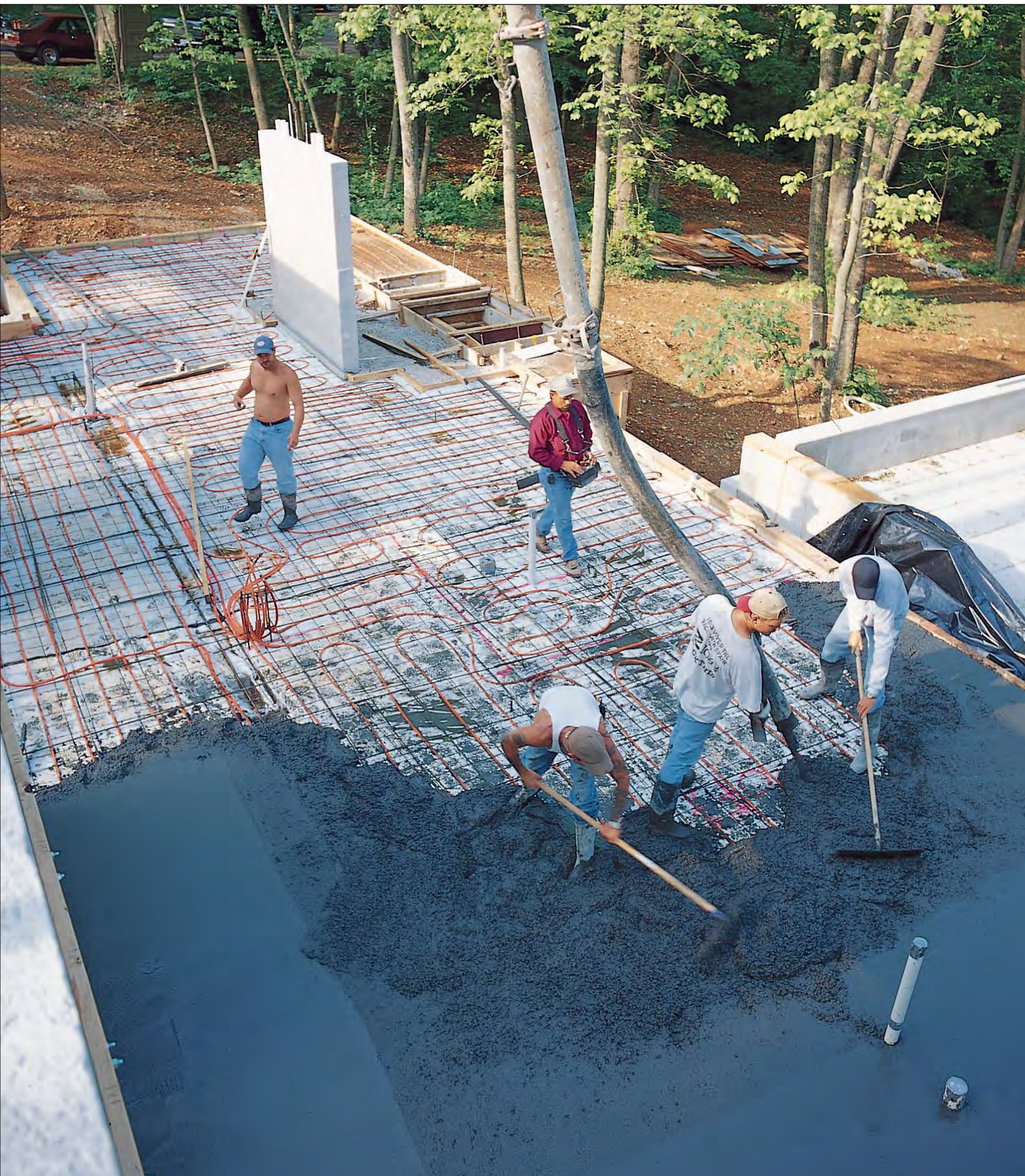
A bird's-eye view of a concrete pour with radiant heat equipment.
