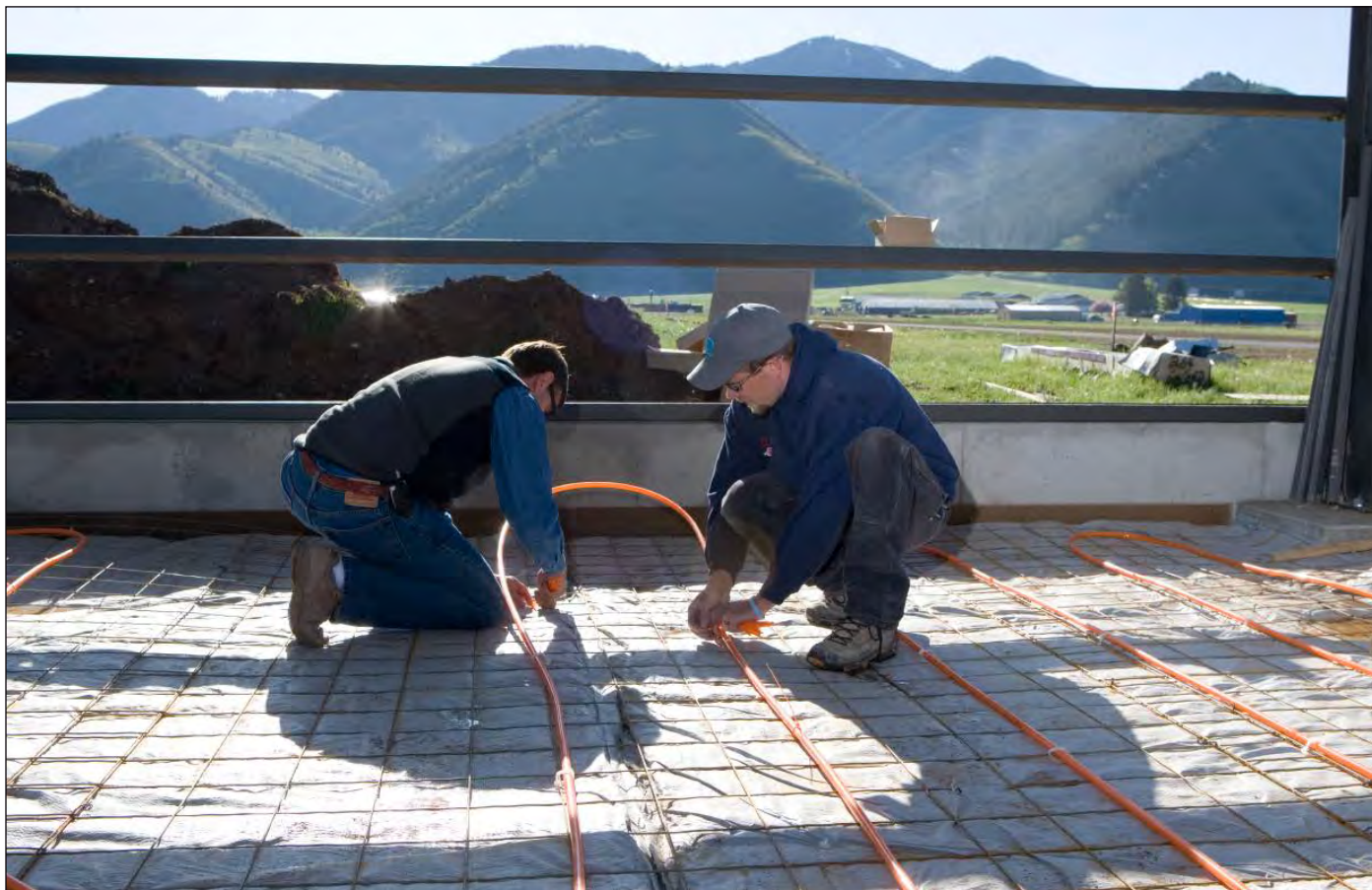
Radiant heat for an interior space that was later covered by stamped concrete.
