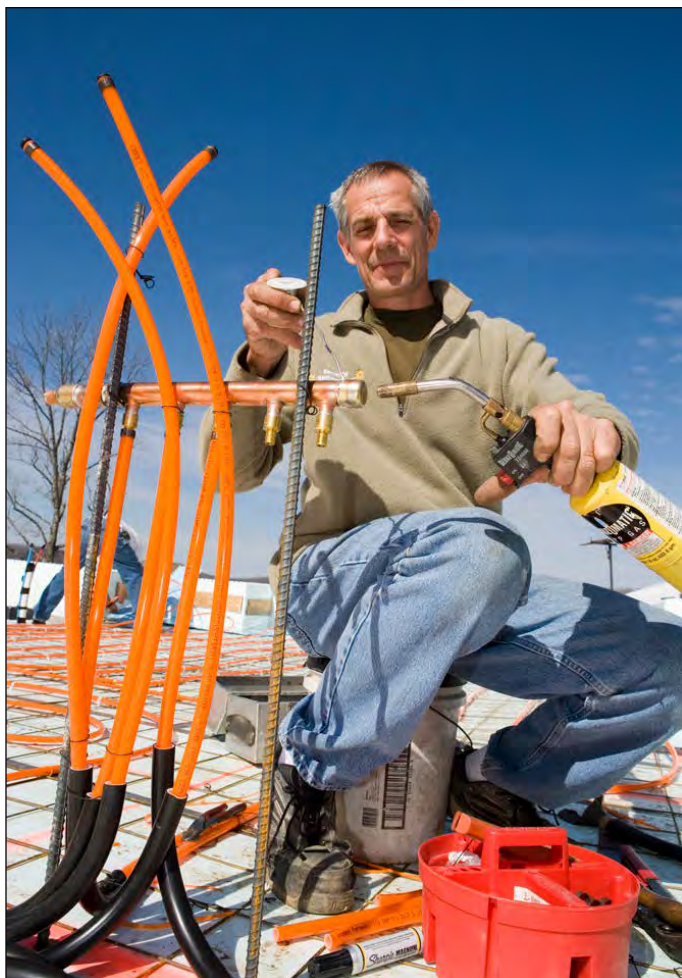
Above Left and Right: Bob “Hot Rod” Rohr installs radiant heat equipment on an under-concrete job in Branson, Mo.
