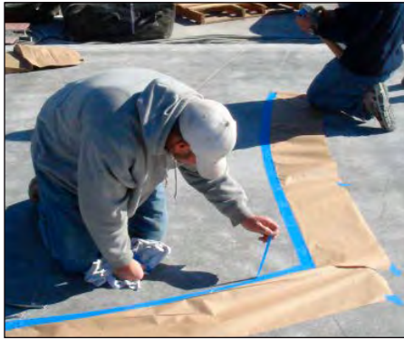
Taping and masking.
