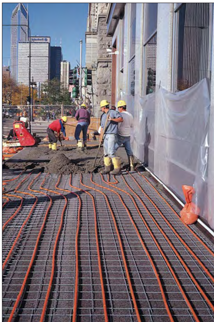
Below: Snow-melt application on a city sidewalk.
