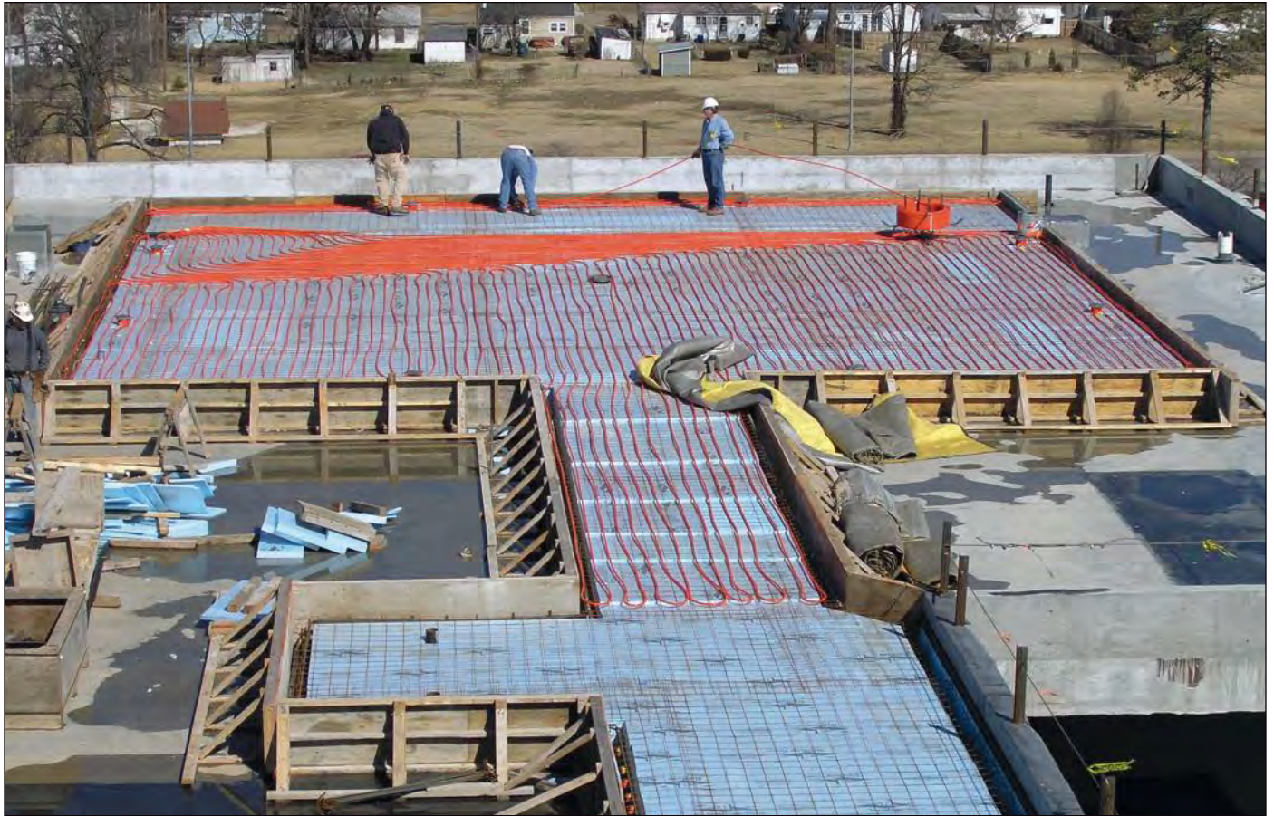
Radiant heat being installed under a helicopter pad.
