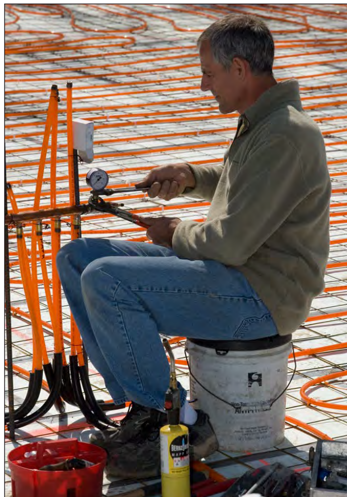
Above Left and Right: Bob “Hot Rod” Rohr installs radiant heat equipment on an under-concrete job in Branson, Mo.
