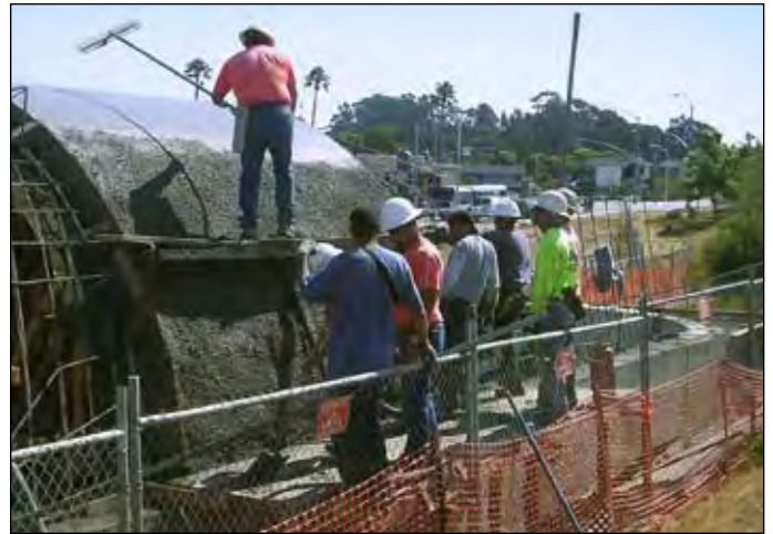
After the shotcrete was sprayed onto the sheet metal covering, crews burned in a “buttery” finish with small fresnos.
