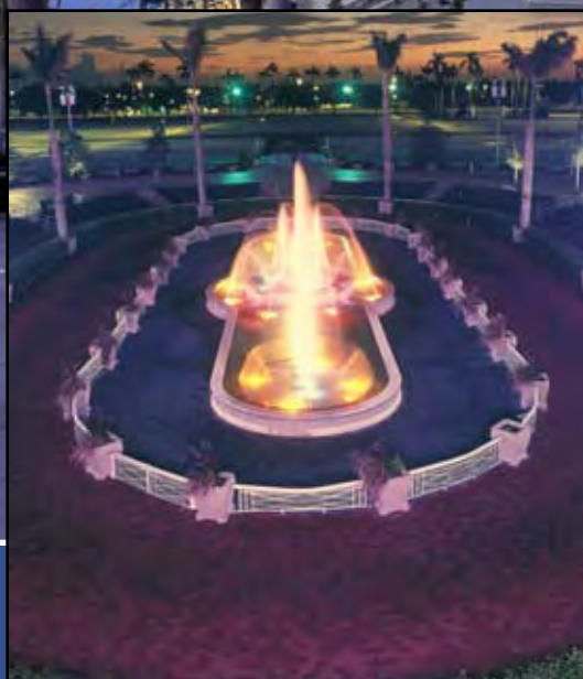
This fountain, located in Gulfstream Park in Hallandale Beach, Fla., is a 2,000-square-foot, cast-in-place concrete structure with cast stone coping and base, hand-painted tiles, and Pebble Tec waterproofing system. Hall Fountains Inc. was the designer and equipment supplier for the fountain, which features a patented real-time music and lighting controller that choreographs the music and lighting with fountain effects.
