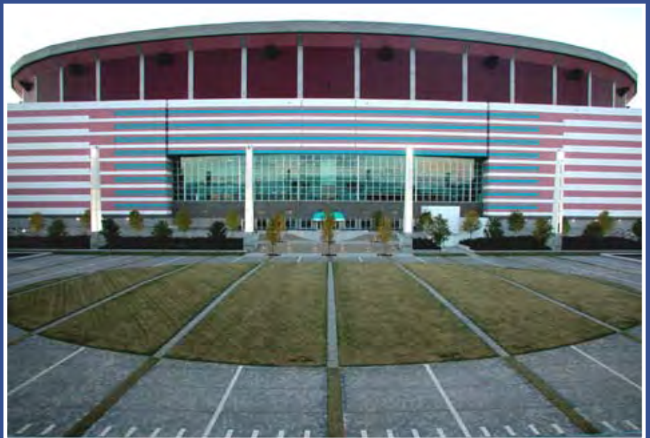
More than 150,000 square feet of concrete unit pavers are used to connect the Georgia World Congress Center to the Georgia Dome in Atlanta, Ga.
