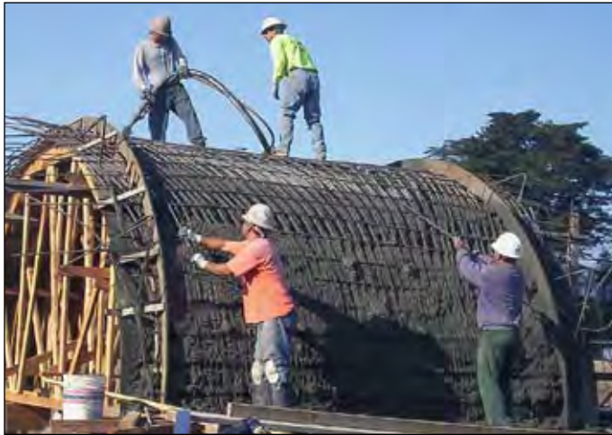
After the shotcrete was sprayed onto the sheet metal covering, crews burned in a “buttery” finish with small fresnos.
