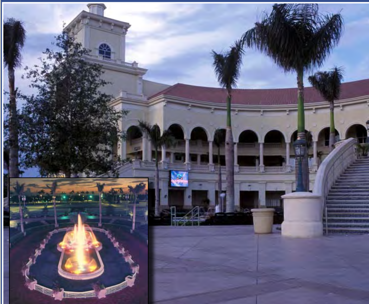
This fountain, located in Gulfstream Park in Hallandale Beach, Fla., is a 2,000-square-foot, cast-in-place concrete structure with cast stone coping and base, hand-painted tiles, and Pebble Tec waterproofing system. Hall Fountains Inc. was the designer and equipment supplier for the fountain, which features a patented real-time music and lighting controller that choreographs the music and lighting with fountain effects.
