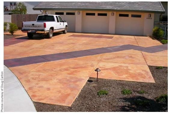
A driveway acid-stained using two stain colors. Notice how splotchy spots show through, even after two stain coats.
