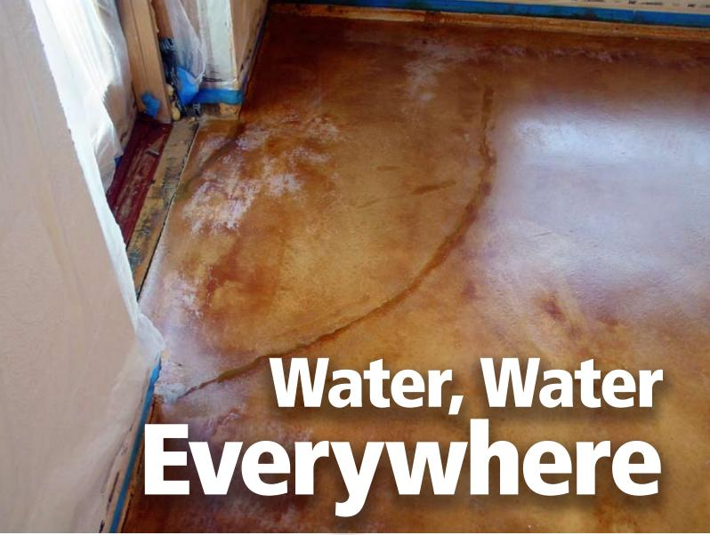
Water that condensed on a stained concrete floor by a cold doorway caused the sealer to white out in the spots where the water pooled.
