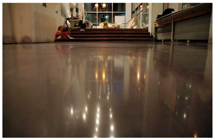
The final floor finish at the Roche-Bobois store in Montreal. It features a semigloss sheen on a restored and colored concrete slab.
