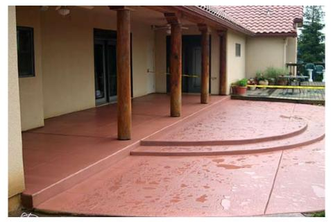
Color sealed with two coats. This method combines the color and sealer, eliminating a step or two. Notice how rain water beads up on the surface.
