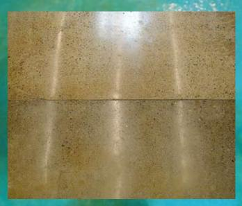
When coloring with dyes or acid stains, only a pre-test will allow you to settle on whether one application or two applications are necessary to achieve your desired color.
