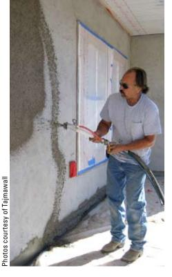
The team at Tajmawall applies shotcrete and pressure molds to the exterior of a house.
