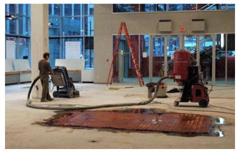
A worker grinds the store floor with low-grit metal diamonds to remove old self-leveling concrete. Water was used to soften the wood flooring prior to its removal by the demolition crew.
