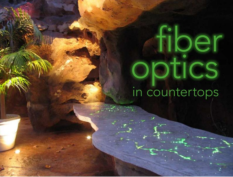
A food-service bar top for an outdoor pool area in Old Westbury, N.Y. Embedded fiber-optic strands create a translucent effect in the concrete.
