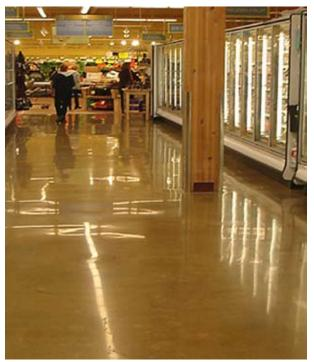
On this project by Seattle-based company Concrete Restoration, the end user desired a cream finish. In order to keep the cream, the floor was finished to to a low flatness level (F(f)), leaving behind a wavy pattern in the existing floor.
