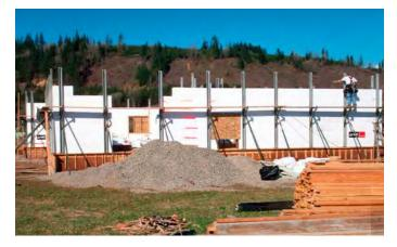
that two built-in layers of foam insulation are installed at the same time. The forms, instead of being removed after the concrete hardens, remain in place and become part of the wall structure, with drywall being the next step.
