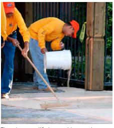
The polymer-modified cementitious overlay installs and dries quickly, so residents were able to continue using the pool each afternoon and evening.
