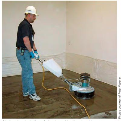
Grinding with a classic MasterCraft swing machine. Note the weights that have been added for increased head pressure.
