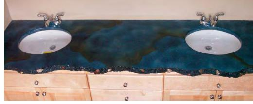
This concrete countertop in the master bathroom features exposed shells highlighted with paint.
