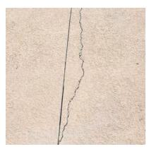
Cracks like this one in the existing pool deck were repaired and old brick-patterned concrete filled in and leveled to provide a new bonding profile for the overlay.
