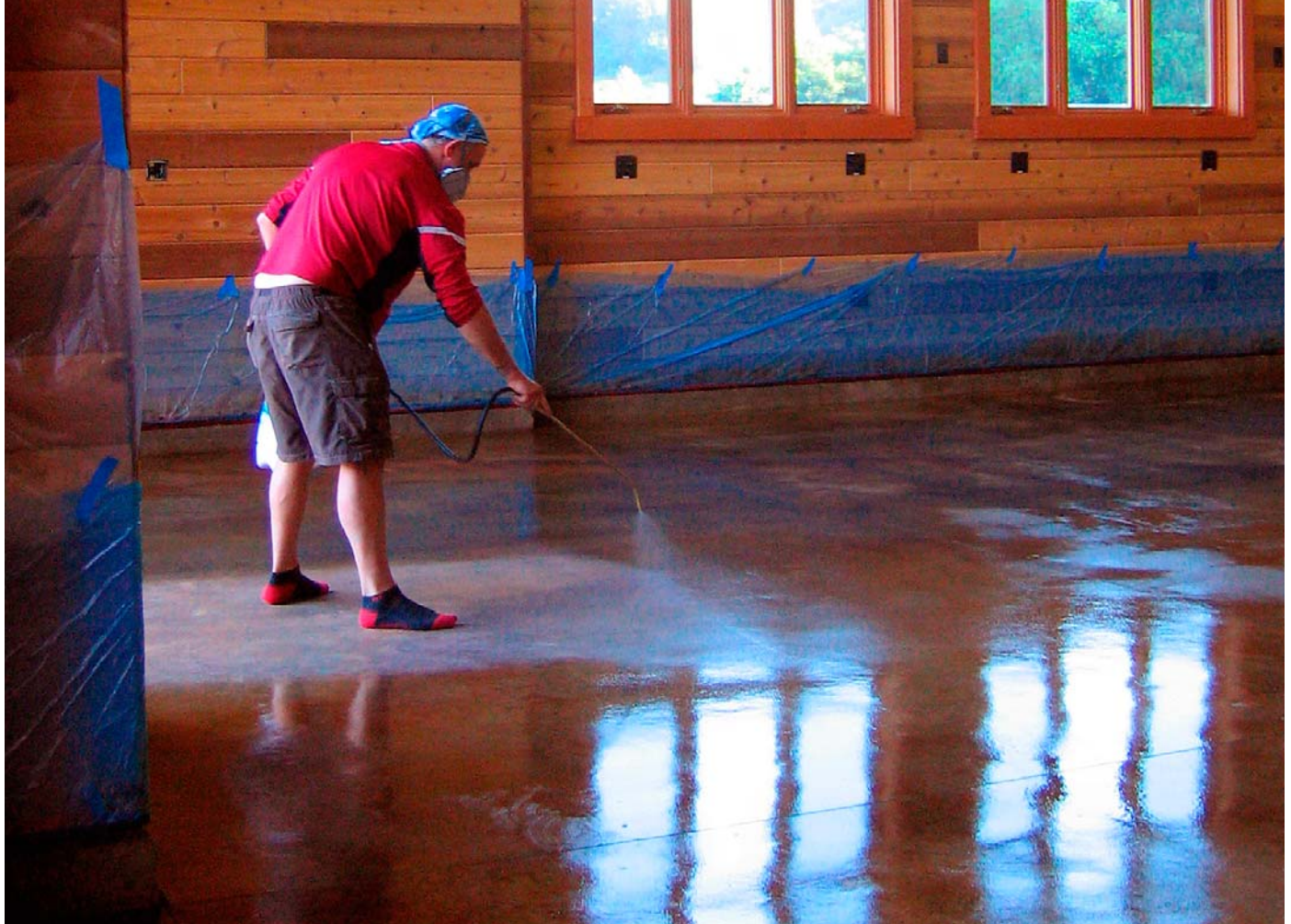
Applying solvent-based acrylic lacquer. Most projects require three sealing coats.
