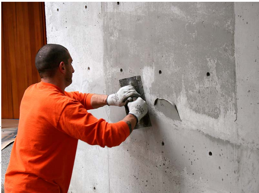
Steve Fox of Seattle's SAK and Patch applies a coat of Raeco's SkimWall in Seattle Gray. The project is a modern residential project whose architect wanted to retain the look of the cast-in-place concrete walls while masking the color variations between pour lines.
