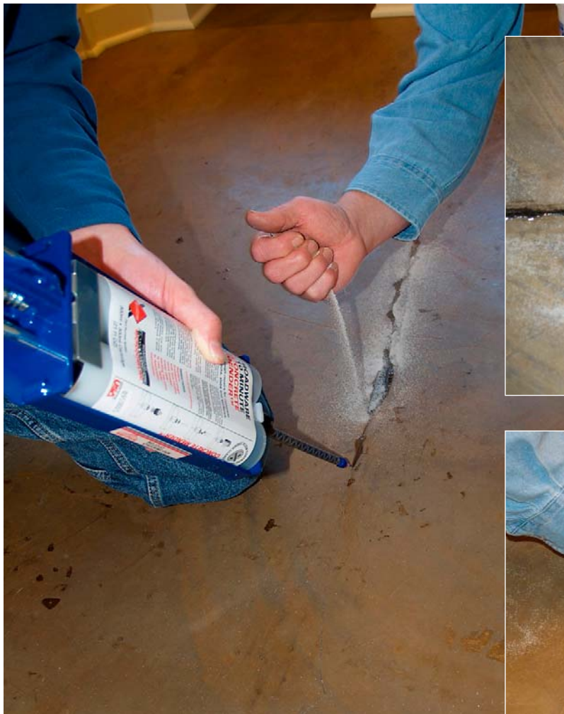
10 Minute Concrete Mender and fine-grade sand are added to hairline cracks on a decorative concrete floor.
