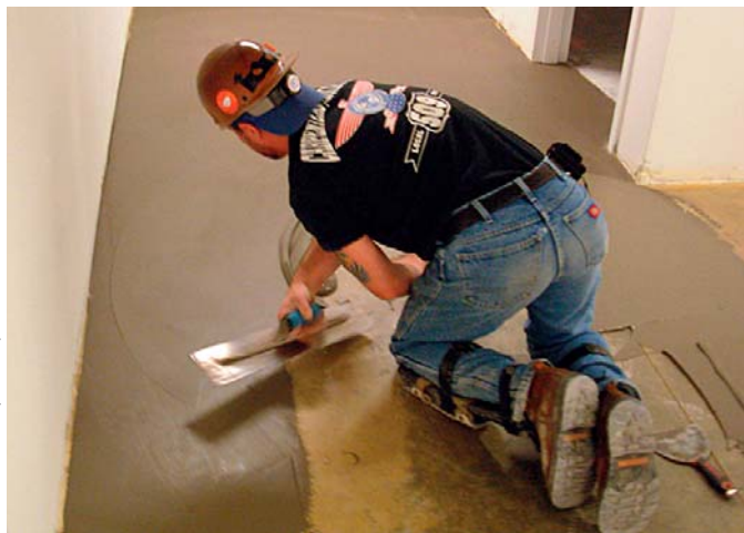
SkimCrete XL, from Dependable Floor Products, is being applied here as part of the company's Moisture Suppressant System.
