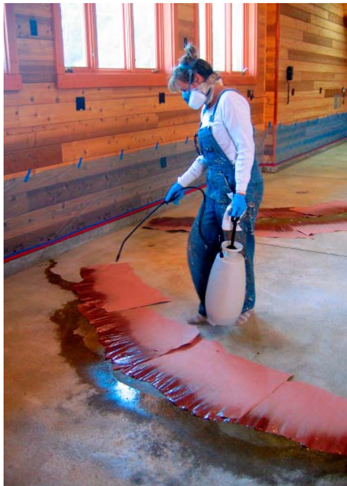
Flashing a stepped-back strata edge. Note the Ironite fertilizer clay granules that have been applied sporadically. The granules "melt" as stain is applied and leave a rusty orange spotting. This spotting is similar to knots in wood.
