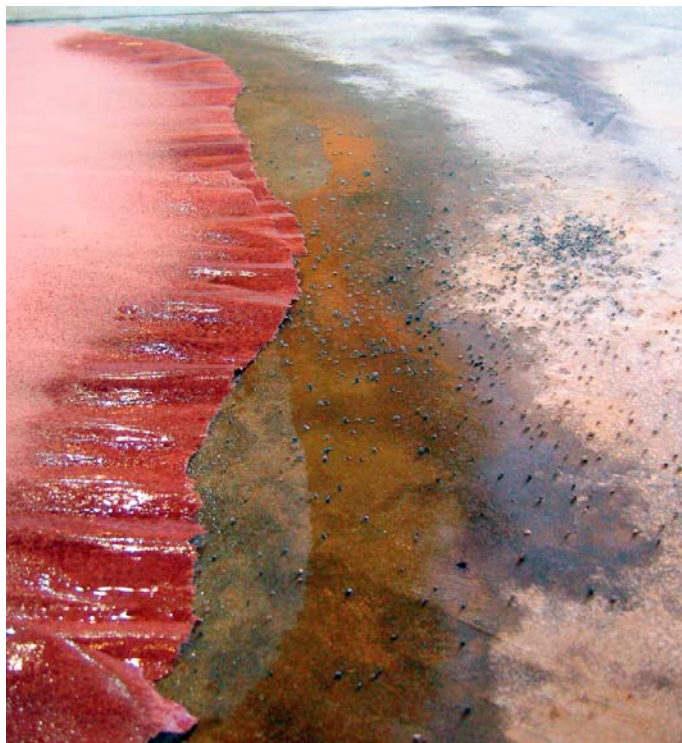
Ironite granules melt and deposit color as acid stain is applied.
