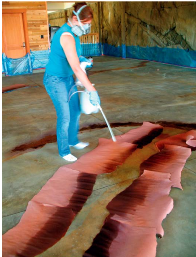
Additional dye strata. This worker is flashing with orange-brown dye to create two hard torn-paper edges.
