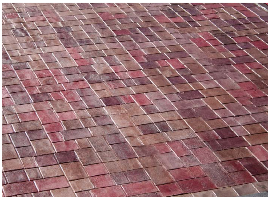
With the help of SureCrete Design Products and Art Stamped Concrete, contractor Craig Heidinger was able to match a stamped overlay to an existing paver pattern used throughout the resort.
