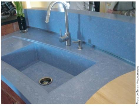
One advantage of using white cement for decorative concrete is that it provides a neutral tinting base and consistent color results. Every color is possible with it, from white and black to blue and pink. This blue sink was created by Concrete Concepts and Design.
