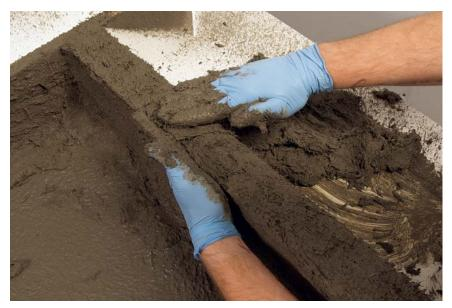
Step 9: Once the scratch coat has been applied, begin the application of the vertical back coat. Starting from the bottom, build the concrete up the vertical wall, holding the wall with one hand and using the other hand to smooth the top. You want to pull the mix over the top of the wall. This helps to keep the vertical back coat from pulling away or slumping.
