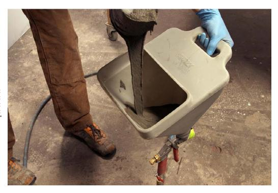
Step 4: Load the hopper with 2 to 3 quarts of the face-coat mix. Turn on the air and do a test spray on a piece of scrap. Set the air flow so the spray is just above "spattering."
