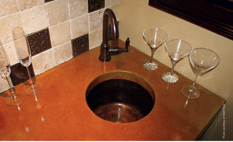
This bar top, created by Matt Hine of Progressive Concrete Coatings, started as a white concrete base and was treated with a custom-blend, multiple-application acid stain. It's been sealed with two coats of a clear polyaspartic coating.
