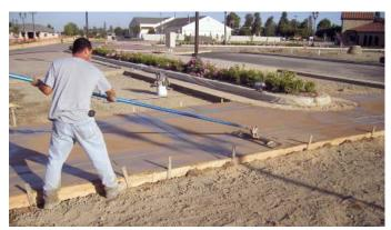
A wood bull float is used to work color into the surface.
