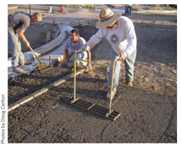
The mix is placed with a low slump and rocks are tamped down.
