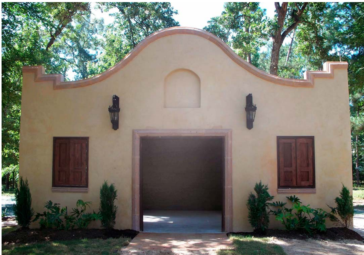
After the chapel was built using a Tradical Hemcrete wall system and lime stucco, it was finished with lime wash.
