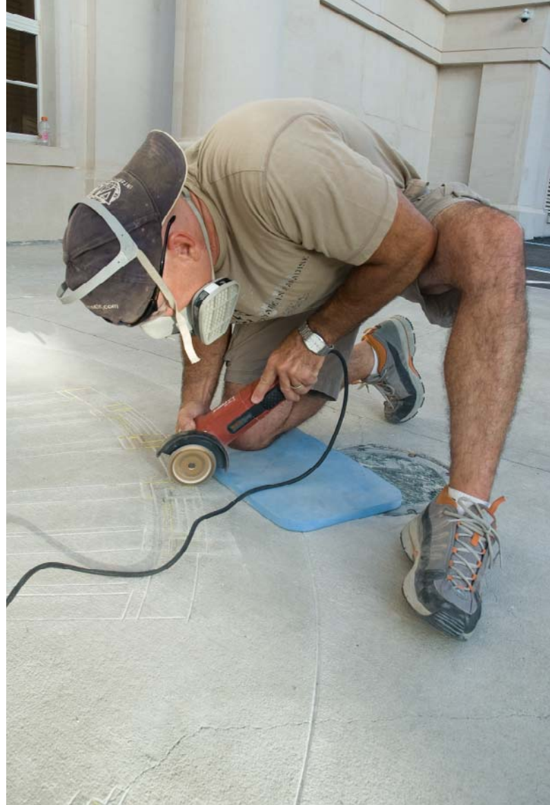
Gerald Taylor scores the design for the Freeman Justice Center project. He is using a crack-chaser diamond blade to create a V-shaped line.
