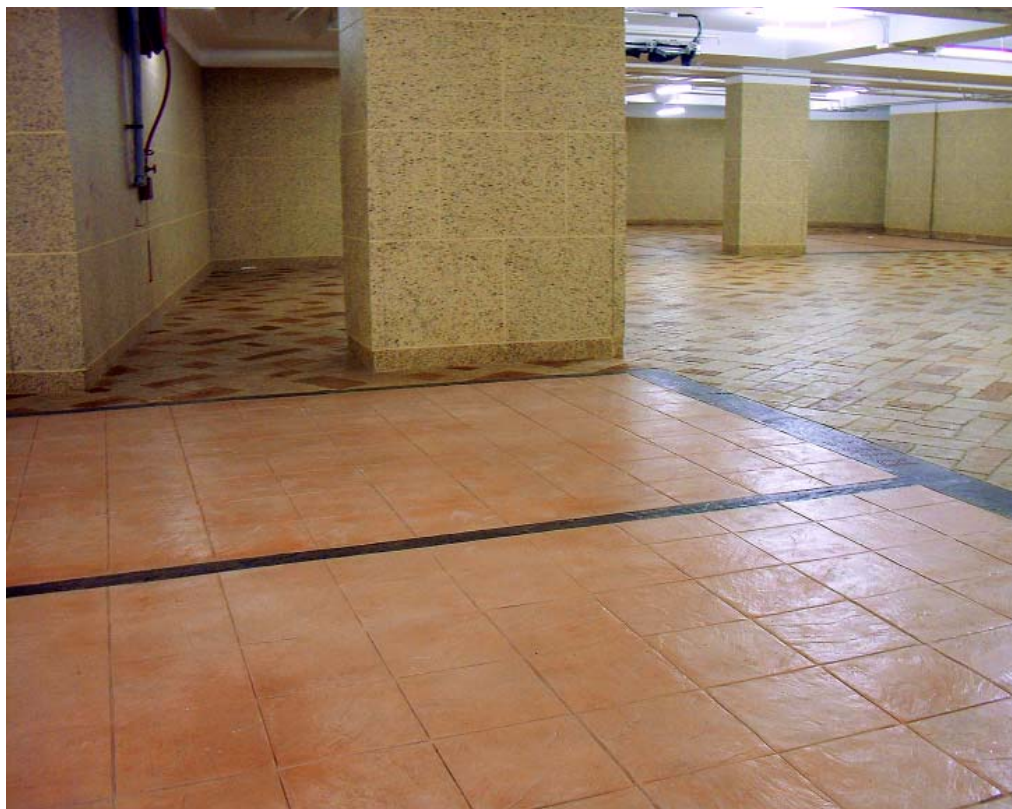
The parking stalls were stamped with Concrete Solutions' Ashlar-Italian Slate 12-inch tiles. The black lines were textured with Italian Slate texture mats, and the driveways with English Fieldstone Large stamps.
