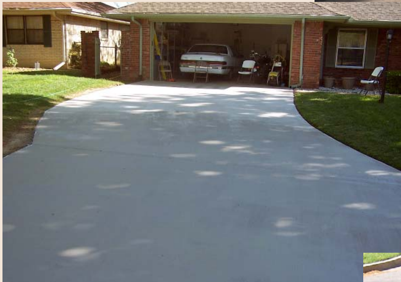
Jerry Van Cleave of VanCrete Decorative Concrete repaired this Tulsa, Okla., driveway using a ductile concrete mix with PVA fibers from GST International LLC. The fibers were used to repair the cracks, and then an overlay was applied.
