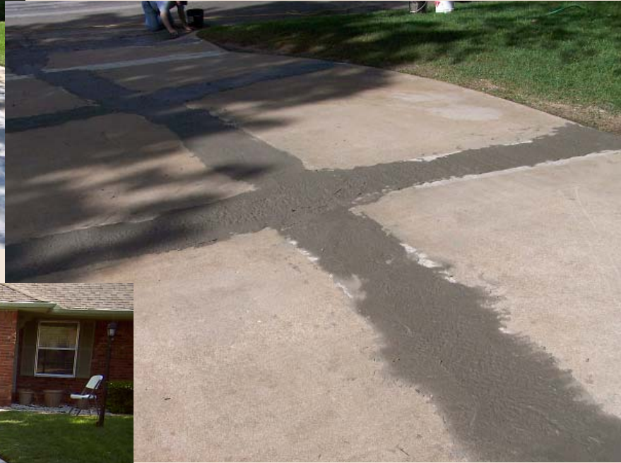
Jerry Van Cleave of VanCrete Decorative Concrete repaired this Tulsa, Okla., driveway using a ductile concrete mix with PVA fibers from GST International LLC. The fibers were used to repair the cracks, and then an overlay was applied.
