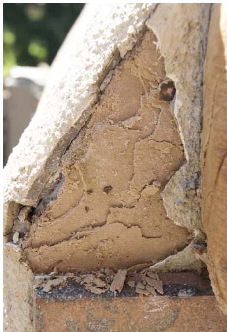
Water and freezing weather caused deterioration of this HardieBacker fiber-cement board.
