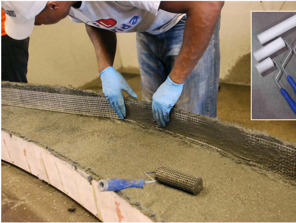
Scrim is being used to strengthen the dropped edges of a 14-foot-long reception desk.
