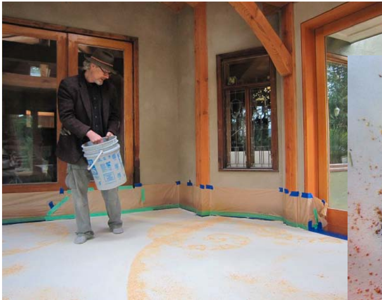
Sculptor and decorative concrete customer Thomas McPhee casts sand and sawdust at his home on Salt Spring Island, British Columbia. The materials will act as a mask, producing graphic edges or variegation in dye washes over this Colormaker Arapido cementitious overlay.
