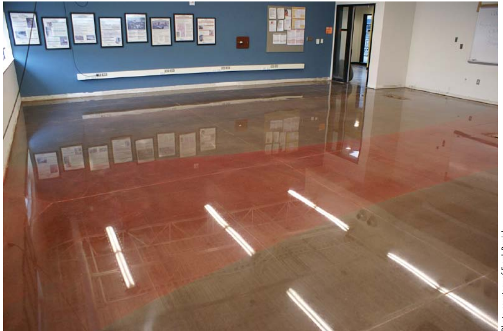
Clark Branum and Frank Benish polished this training-classroom floor at the Western Washington Masonry Trades training center in Seattle. The floor demonstrates high gloss and high clarity. The slip coefficient is 0.74.
