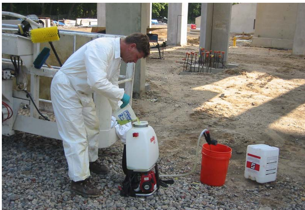
A Tom Ralston Concrete crew member fills up a gas-powered sprayer for acid staining.
