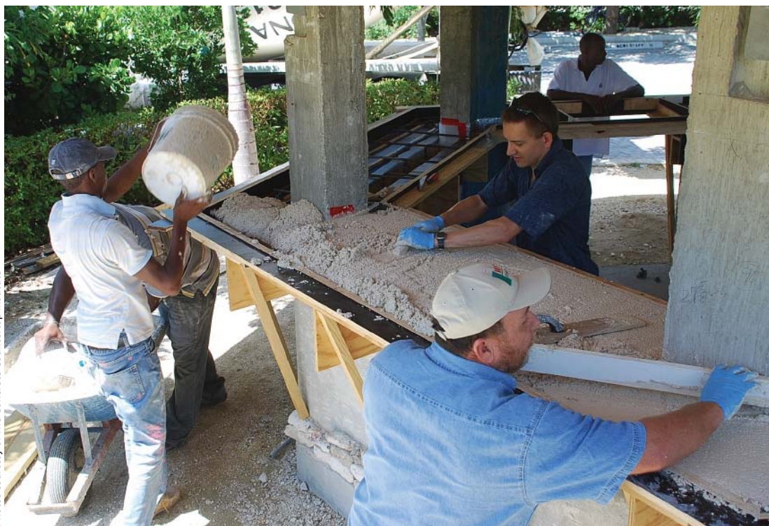
Jeff Girard (in the dark blue shirt) helps a crew place and screed concrete for a bar top in the Cayman Islands.
