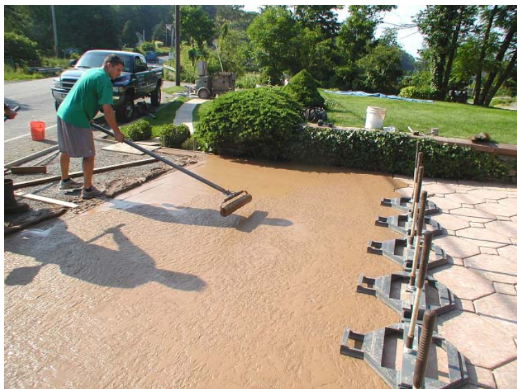
Timothy Fisher applies texture using Unique Concrete's custom-made roller.
