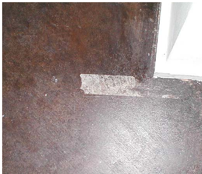
Another acid-stained, sealed floor damaged by painter's tape.
