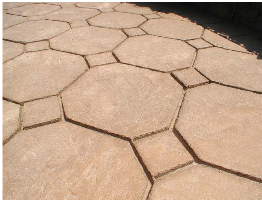
Larger voids allow the use of enough grout to withstand severe freeze/thaw cycles.
