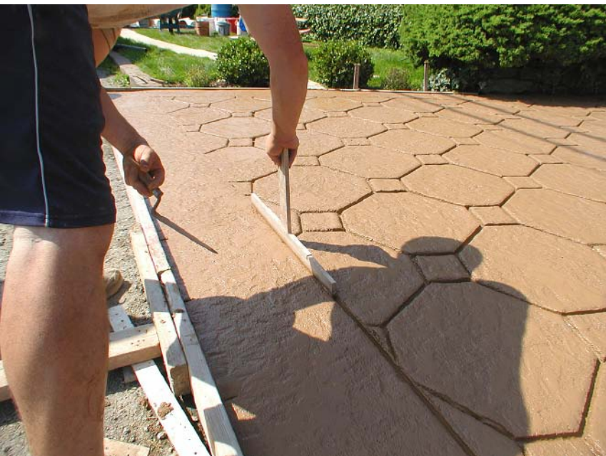
When hand-chiseling borders, you can create custom border shapes and sizes.
