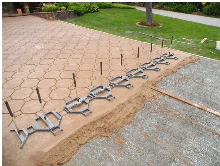
Custom-made "cookie cutter" stamps designed and fabricated by Barry Fisher.
