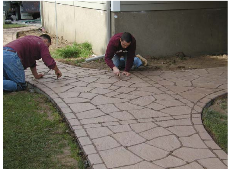
Travis and Timothy Fisher tool the grout once it is at a proper consistency.
