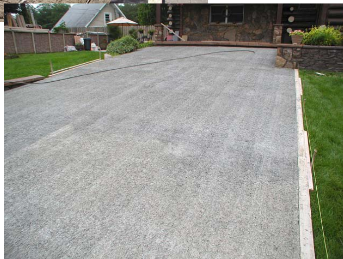
This slab was scarified to create a mechanical bond for the layer of decorative concrete to grip.
