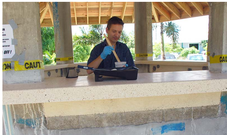
Jeff Girard mixes sealer to coat the finished cast-in-place bar top.
