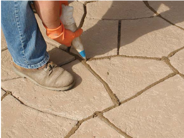
Polymer-modified grout is applied using a traditional masonry grout bag. Grout can be any color or left uncolored for a traditional look.
