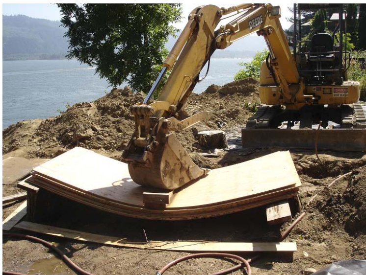
To bend plywood into curves for the form, stack of the material were soaked in water, forced down with a track-hoe bucket and held in place overnight.
