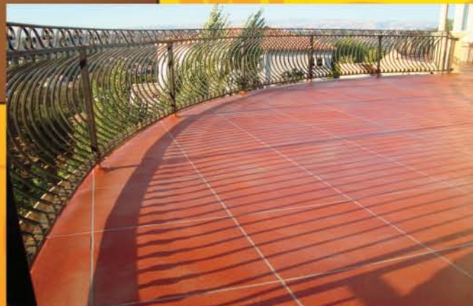
Versa-Crete Tile Finish over a Wood Deck Installed by GM Coatings
