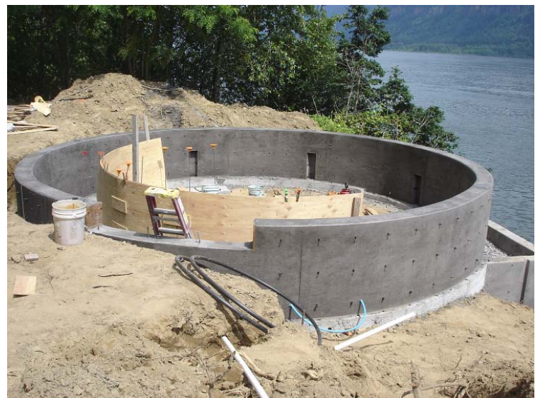
The circular wall was poured 10 inches thick, using 3,500-psi concrete mix colored with Davis Colors’ Chameleon Mix-Ready dye system in Pewter.
