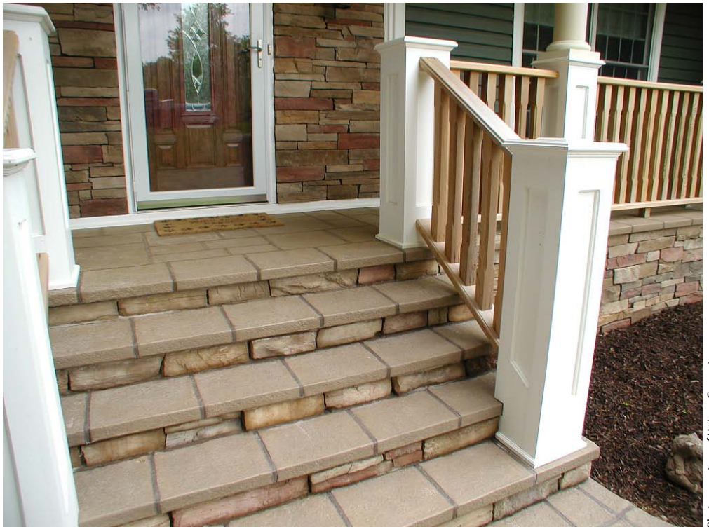
This West Milford, N.J., home has more curb appeal thanks to a cast-in-place overlay system over a wood deck.
