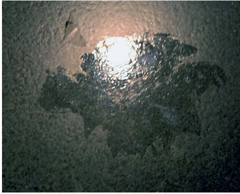
In this photo, the matte layer of a sealer has peeled off to reveal the shiny undercoat.
