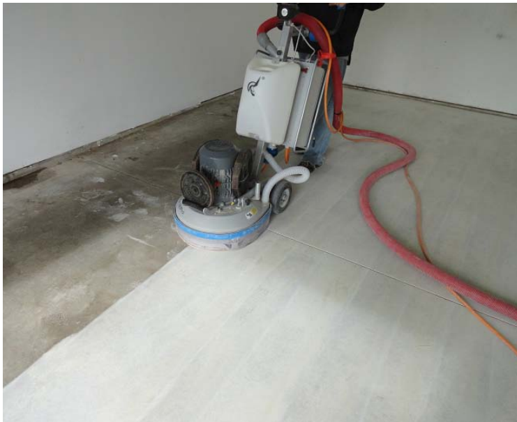
Using a Lavina 20N machine, a Dancer Concrete worker grinds the surface to remove the top layer of cement and contaminants.
