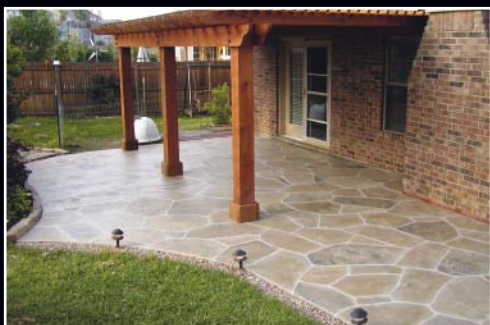
McKRETE™ DRY MIX & ADDITIVE Indoor or outdoor, this user-friendly acrylic material can be stenciled, taped or textured.
