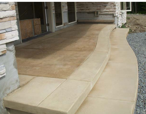
Color hardener was used to make this step border a lighter shade of color than the placed concrete.
