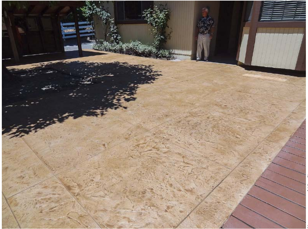
This Santa Rosa, Calif., patio was previously a series of concrete slabs and pavers. After the pavers were removed and new concrete was poured between the older slabs, Concrete Staples were used to join new and old.
