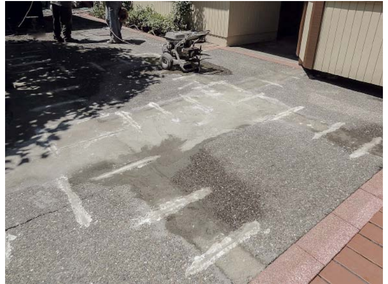
Concrete staples combine the new and old concrete.
