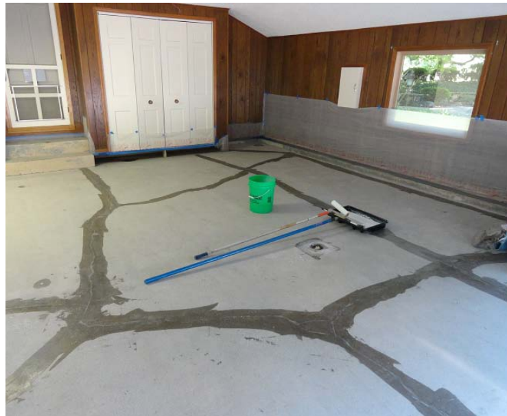
Addressing cracks is part of any professional floor install. Help your client set expectations regarding why concrete cracks and how you will repair it.
