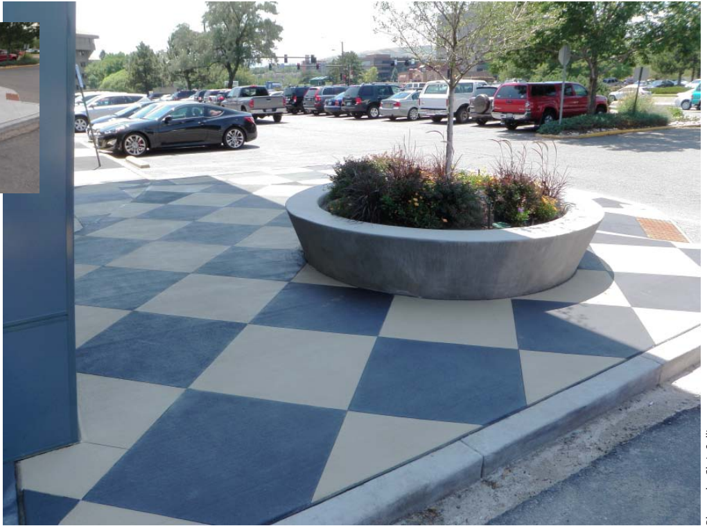
Above: Pritchard Concrete, Golden, Colo., colored concrete at this Lakewood, Colo., shopping center using epoxy-based ReStore Solid Color Stain from Helix Color Systems in Stone Gray and Latte. Top left: Before the work.
