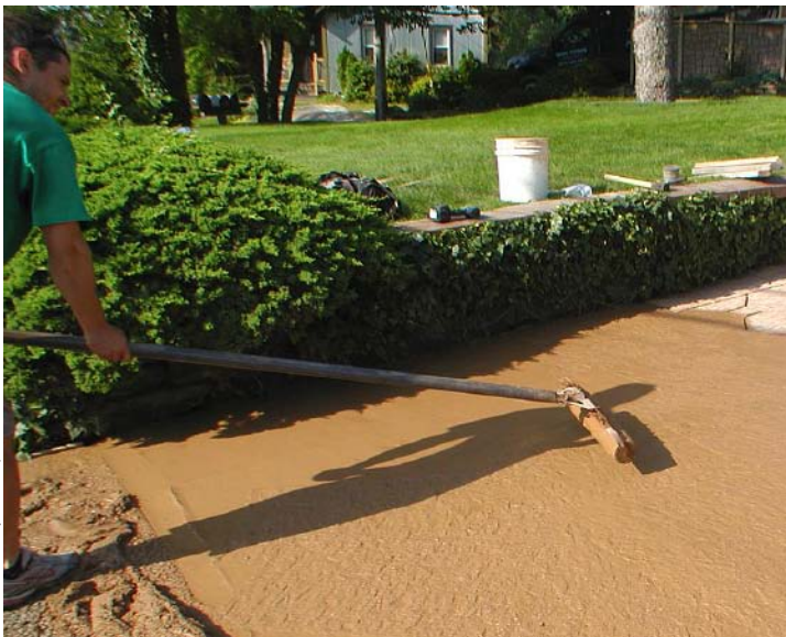
Above: Texture being applied to a slab with a textured roller.
