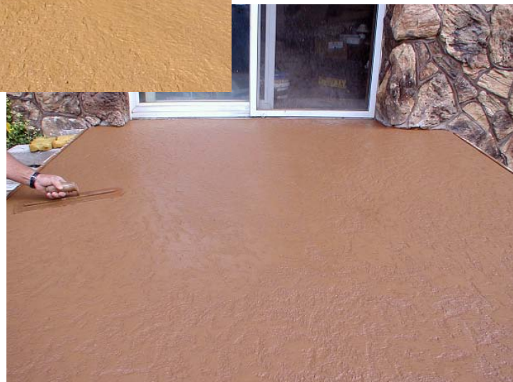
Right: The knockdown of a texture, done with a trowel by hand. The applicator can control the degree of knockdown.
