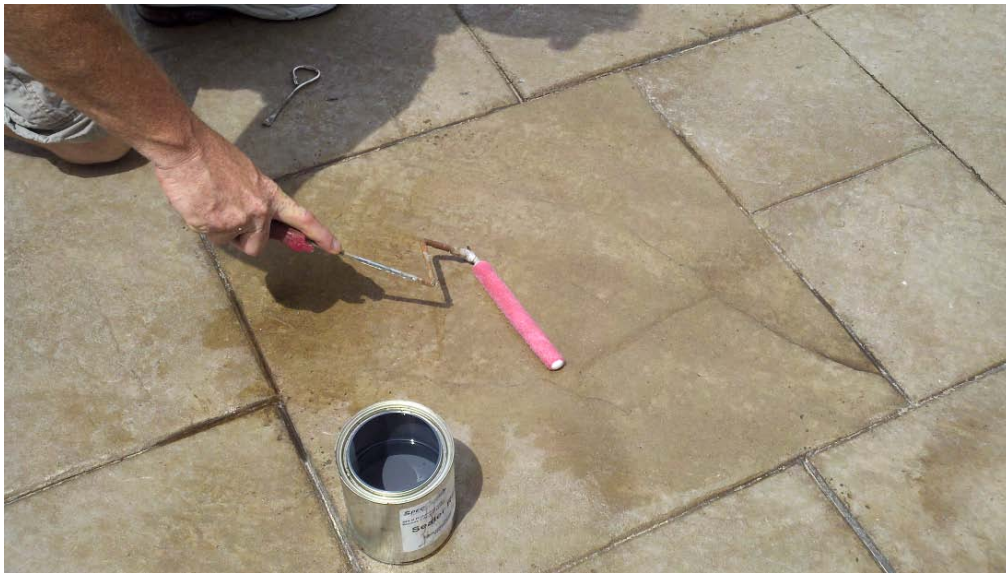
Rolling xylene on a dull and blushing sealed concrete surface can help clear the sealer and bring back the luster.
