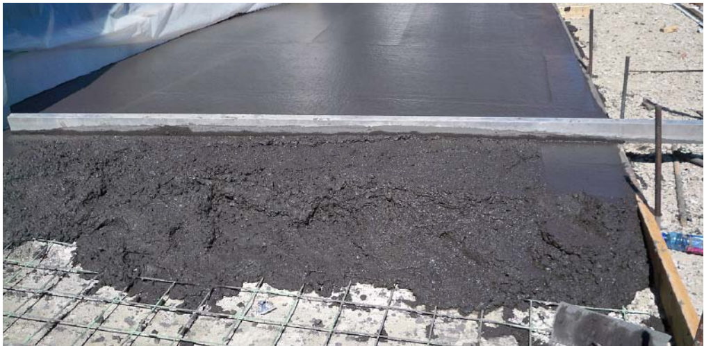
An L. M. Scofield Chromix Admixture in C-34 Dark Gray was used to achieve long-term color durability for a high-traffic area on a dock at the Intrepid Sea, Air and Space Museum, New York City.
