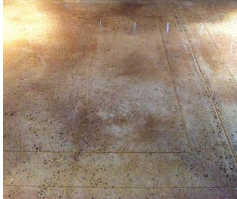
Above: The color-troubled polished concrete floor in a residential basement, before a four-step process fixed the problem.
