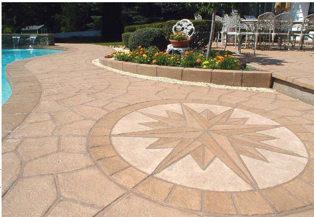
This resurfaced pool deck and patio in Lake Hiawatha, N.J., features Unique Concrete NJ's custom-made field stone stamp and medallion. The integrally colored concrete was stained with a homemade water-based system and sealed with Kingdom Products' Kingdom Cure, a high-solids solvent-based sealer.
