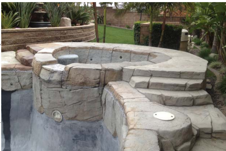
This residential project in Rancho Cucamonga, Calif., included a complete restoration of the rock pool and spa. Kevin Brown of KB Concrete Staining, Mira Loma, Calif., used NewLook materials for the renovation, including the company's SmartColor stain in Milk Chocolate, White, Black and a tan shade.
