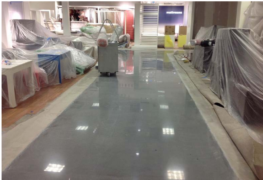
Each night, the merchandise is covered before work can begin on the "streets" in this JCPenney store at West Towne Mall in Madison, Wis. This particular job features CTS Cement's Rapid Set TRU overlay.
