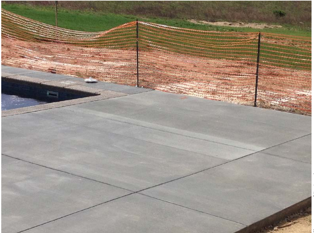
Excess water from a wet broom created this light-colored area on an integrally colored broom-finished pool deck.
