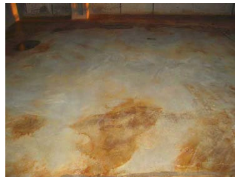
A hard-troweled floor after the acid stain was cleaned off. The blotchy finish is the result of a lack of penetration and reaction on the part of the stain.
