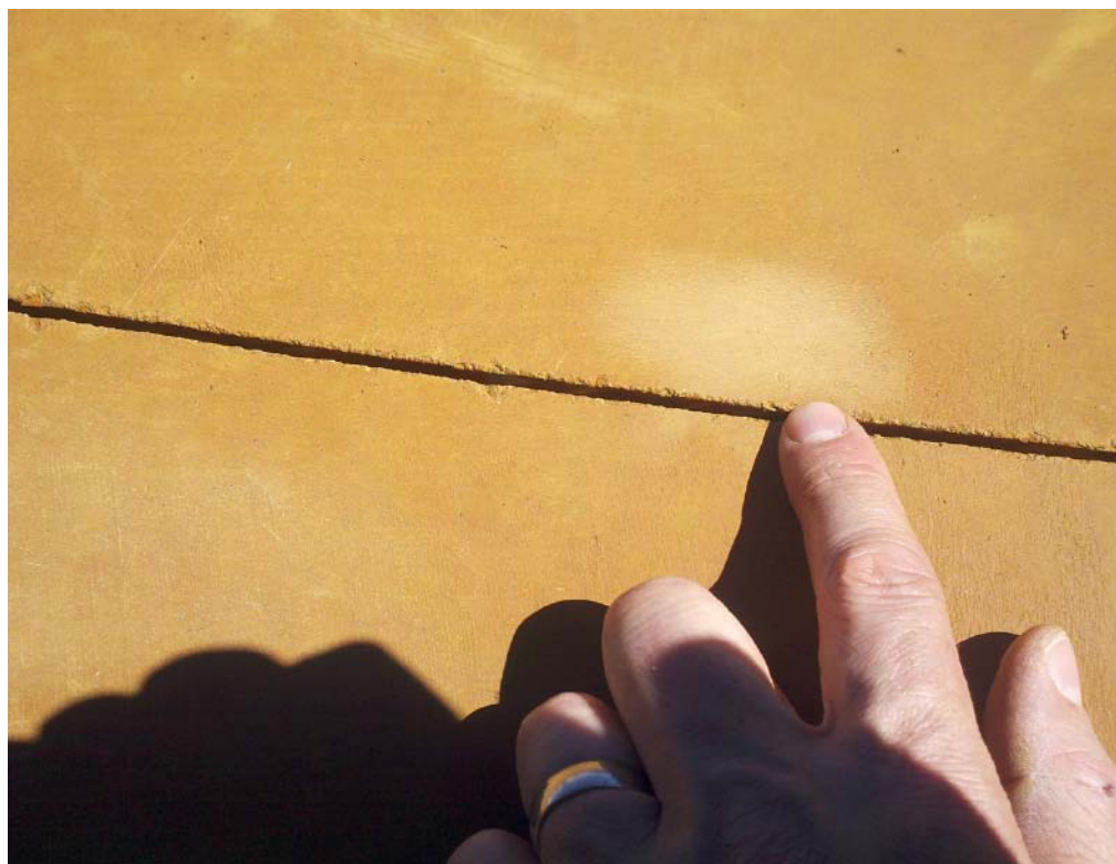
Above and below: Acid stain dusting off the surface prior to sealing due to lack of penetration and reaction.
