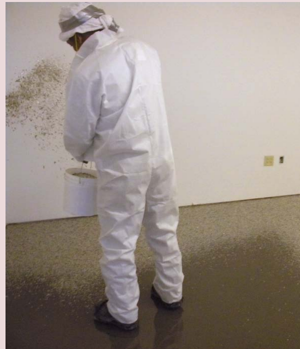
Left and above: Crew members for Nashville-based Fuller Industries Inc. install a mica chip floor at a Nashville book and CD store using mica chips from Torginol and Florock polymers.
