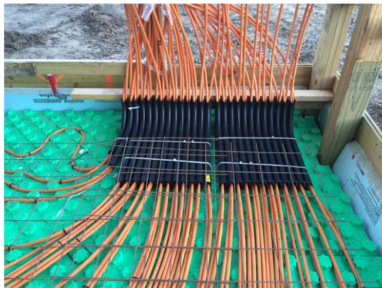
Before Reuben Keim's Ohio-based crew poured a 25,000-square-foot slab for a commercial building in October, a plumber laid out this hydronic tubing on Crete-Heat, a foam board with knobs that hold the tubing in place. Reinforcing mesh is laid over the tubing.
