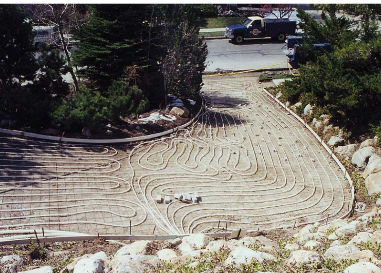
Hydronic tubes solve the problem of removing snow on steep driveways, such as the driveway at this Salt Lake City house.
