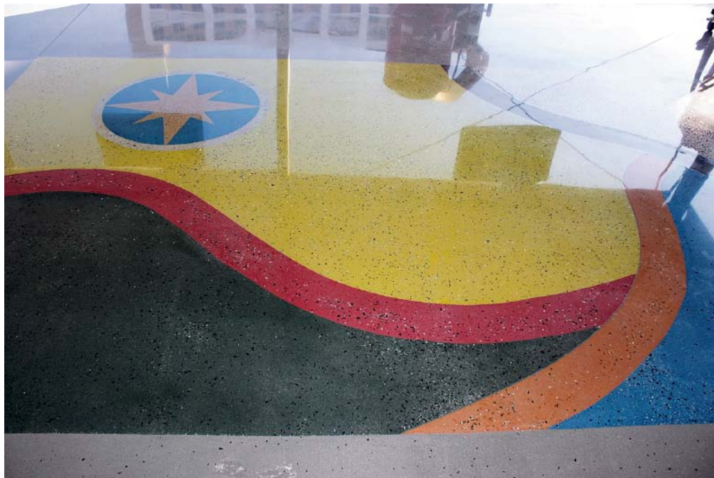
Glass aggregate was mixed integrally into this demo slab for a booth at the 2013 World of Concrete.
