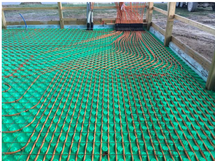
Before Reuben Keim's Ohio-based crew poured a 25,000-square-foot slab for a commercial building in October, a plumber laid out this hydronic tubing on Crete-Heat, a foam board with knobs that hold the tubing in place. Reinforcing mesh is laid over the tubing.
