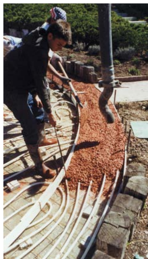
Hydronic tubes solve the problem of removing snow on steep driveways, such as the driveway at this Salt Lake City house.
