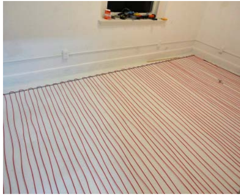
Michele Pondi-Salik, of Davinci Pavement Design LLC, Stratford, Conn., installed a Warmzone radiant heating system in this interior.
