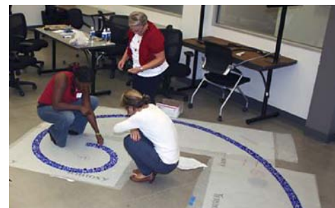
Milena Sellers-Phillips (left) and Maria Keever (rear) add personal touches to the mosaic Fibonacci spiral as Amanda Klemaske Conahan looks on. In the LithoMosaic system, the mosaic is created off-site on mesh, then embedded in the concrete. The mothers placed the mementos on the mesh right side up, and Conahan turned them upside down before gluing.
