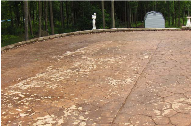
A driveway in Mountain Top, Pa., with salt damage. This property was right off an interstate and the owners tracked salt from the highway onto the drive. Perhaps the concrete was a lower-grade mix or suffered an improper amount of air entrainment at the time of pour. You can see it was not durable.
