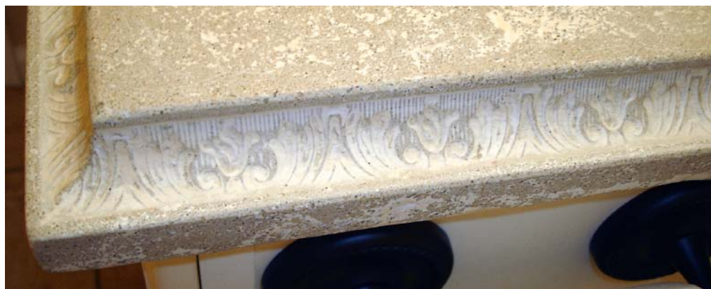
This floral edge is easy (and profitable) to do with concrete, but nearly impossible to get with granite.
