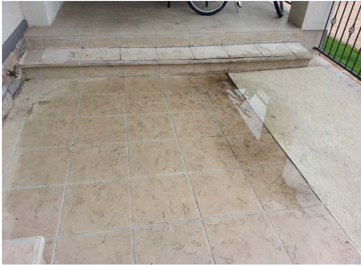
Water pooling on the surface, caused by a rotted and collapsed wood subfloor.
