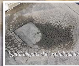
Finished patch applied directly over broken asphalt surface
