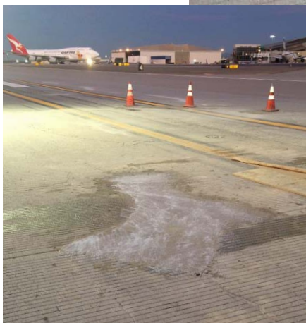
Left: The repair after the work is done, with curing compound visible on the patch surface.
