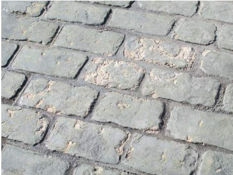
Left: A Nuangola, Pa., driveway with salt damage. Right: The driveway restored with Kingdom Products' Top Cap overlay custom-colored to match the original project.
