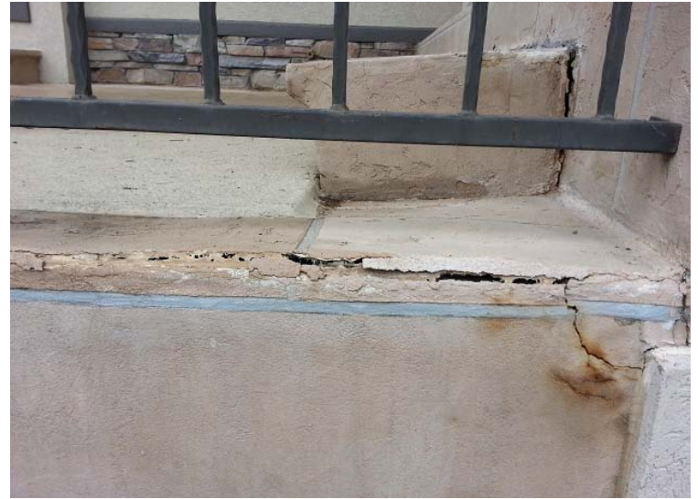
Water intrusion causing failure around the steps.
