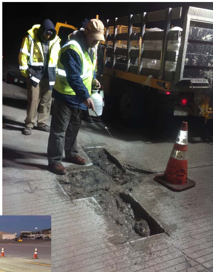
Above: Spraying on a trowel aid for a full-depth repair of an active runway at Los Angeles International Airport.
