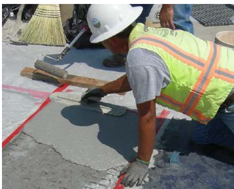
Replacing a failed stamped overlay on a utility access door for the Roseville, Calif., city hall.
