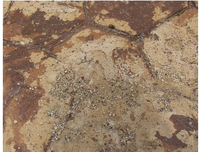
A driveway in Mountain Top, Pa., with salt damage. This property was right off an interstate and the owners tracked salt from the highway onto the drive. Perhaps the concrete was a lower-grade mix or suffered an improper amount of air entrainment at the time of pour. You can see it was not durable.
