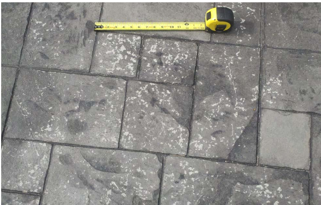
Failing acrylic sealer on stamped concrete near a pool at a private residence in Knoxville, Tenn.
