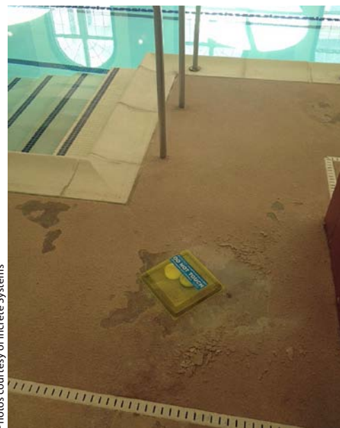
A sealed overlay near an indoor pool at a retirement home in Virginia Beach, Va. It performed at first, until the chlorine pool was changed to salt water. Within months, the topping started to delaminate.
