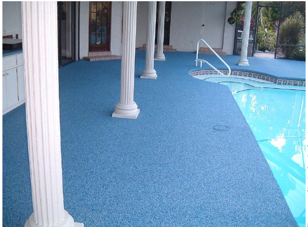
Florida homeowners opted to resurface a patched and repaired concrete pool deck with TPV rubber.
