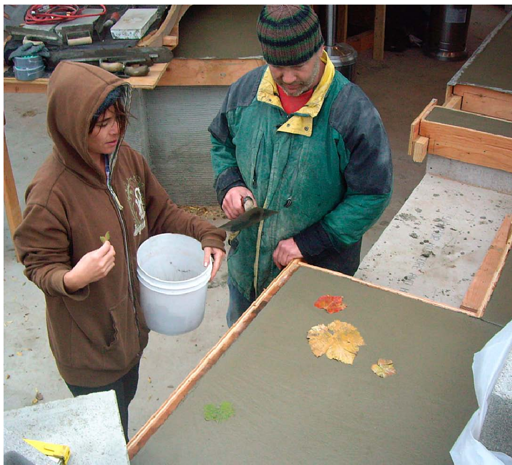
Concretist Emily McClintick art-directs finisher Michael Todd as to the best “random” troweled grape leaf locations. Note the tooled contraction joints at re-entrant corners on counter. The sculptural bar wasn’t jointed.
