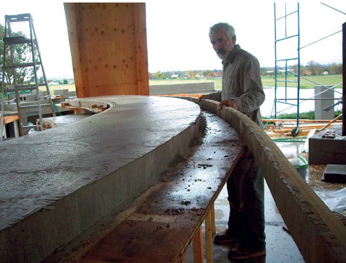
Greg Stanley removes bar forms. Notice the texture, similar to that of a coopered wine barrel. The concrete wasn't edged. Sharp corners will be eased with soft diamonds on a polisher.
