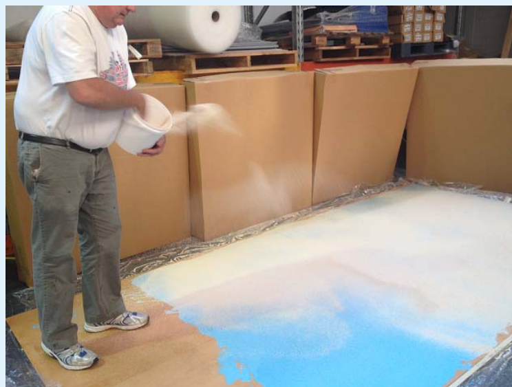
In this demonstration, a man applies a flexible epoxy to a surface and then broadcasts PolySoft microgranules over the top.
