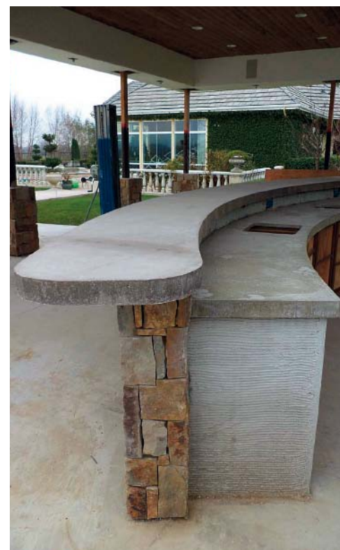
The sculptural bar top is integrally colored and unjointed (a big risk). The countertops are natural gray with "fossil" leaf impressions and minimal joints, at or near blockouts, to control cracking and curling.
