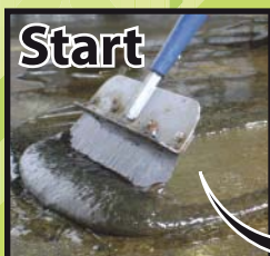
Urethane sealer on concrete floor
