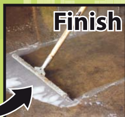
Urethane sealer on concrete floor
