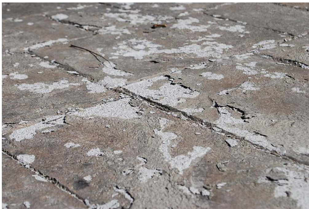
This stamped concrete patio in Louisville, Kentucky, was damaged in the most recent harsh winter.
