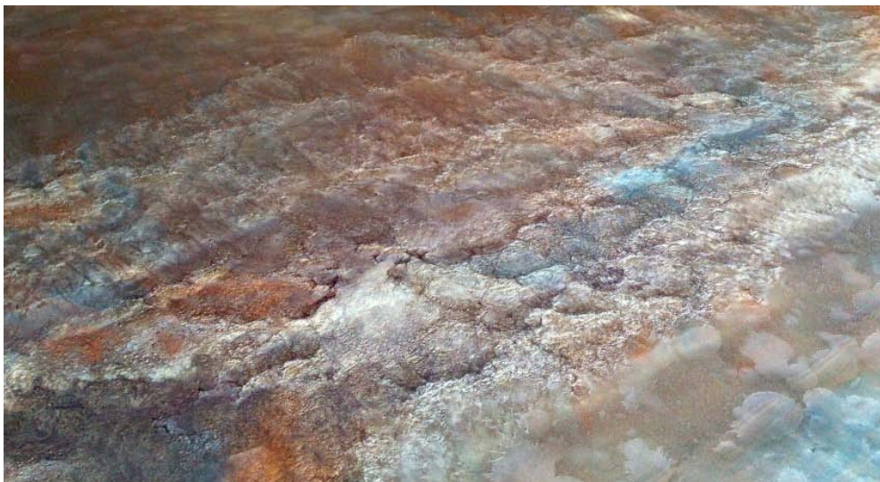
A leaf blower was used to manipulate the metallics and create this look. No solvent effects were applied.
