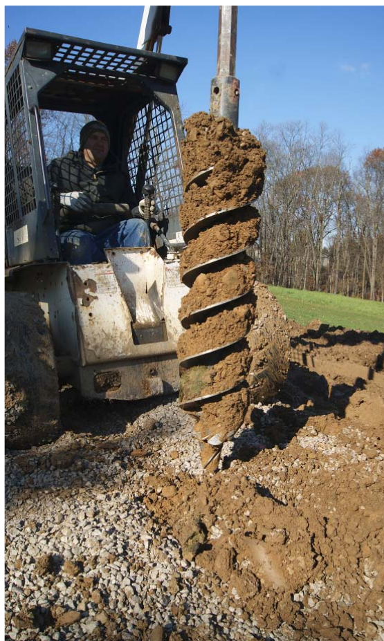
Above: When you see chunks of sod in the dirt on your auger, you know you're down to virgin dirt.
