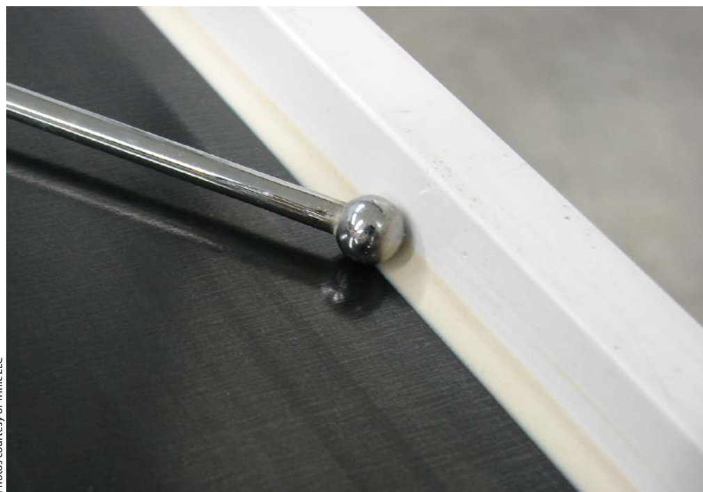
Perfect caulk joints in a variety of radii are possible with clay caulk.
