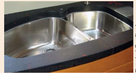
The redone top, with sink bevel revealed.
