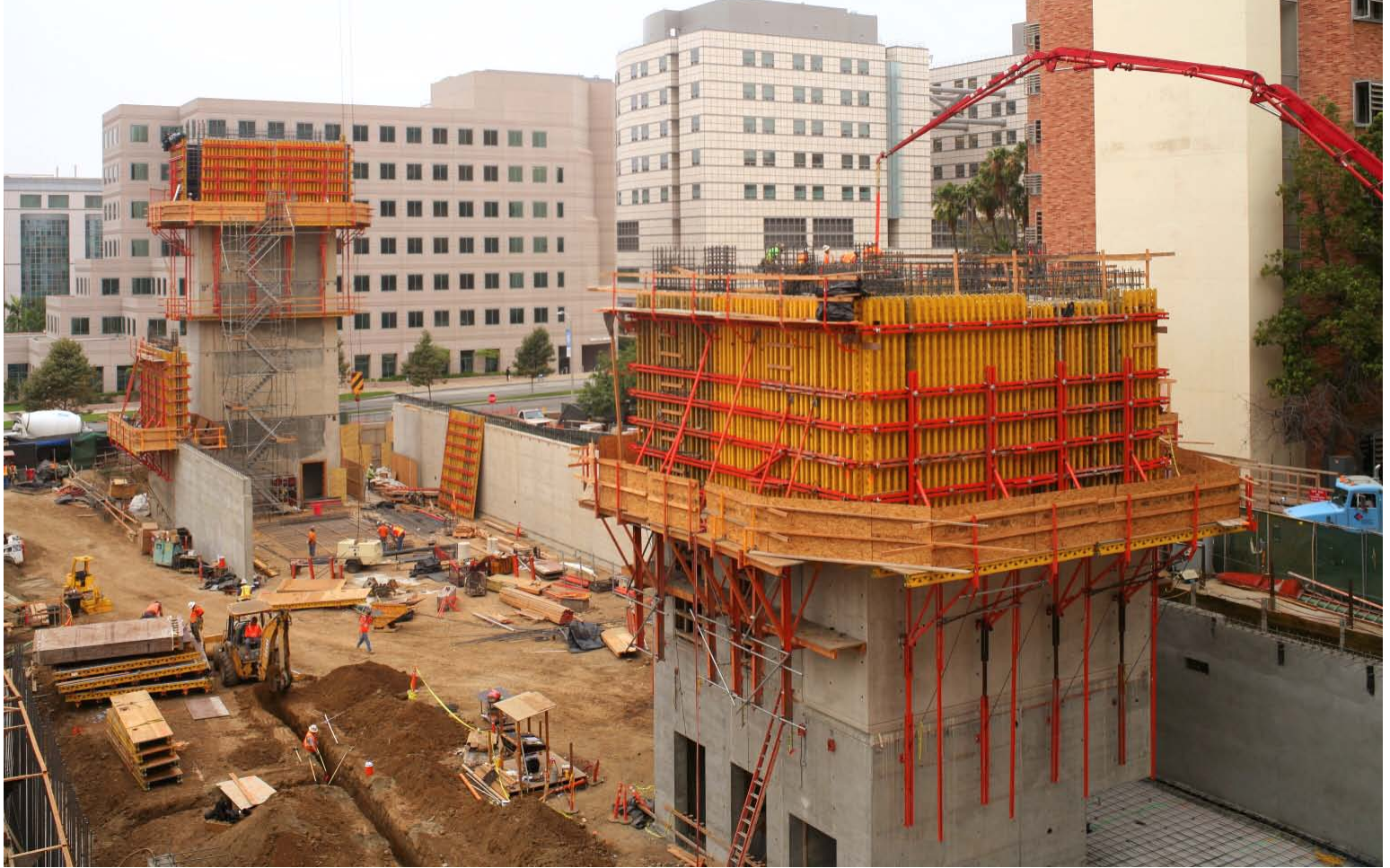
The Wasserman Building is anchored at its east and west ends by tall, massive architectural concrete core towers. Seen here are form work panels in place for a pour. Architectural concrete, including white type II/V portland cement with black, yellow and red color additives, was only used on the exposed components.
