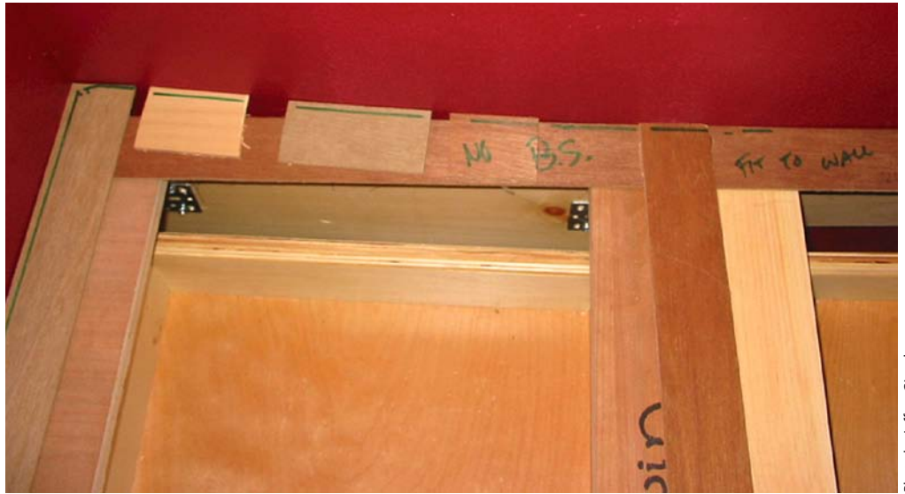
Template with tabs that was created to fit a very crooked wall and corner.
