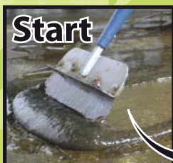
Urethane sealer on concrete floor
