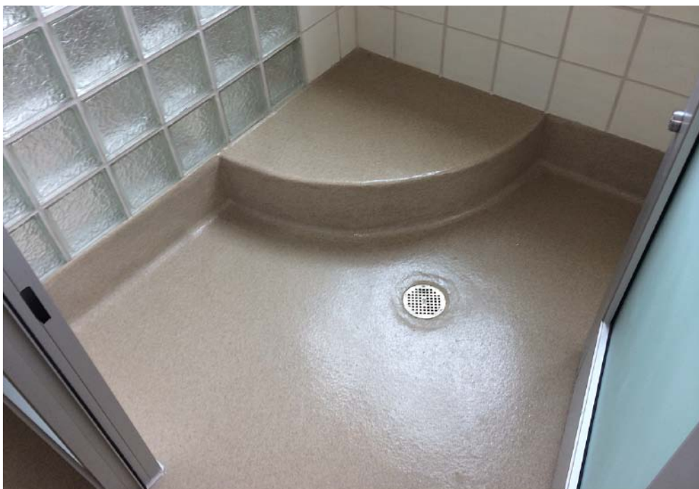
A broadcast-quartz floor by Baltimore-based Durex Coverings Inc. that incorporates the Mosaix Floor system mixture of ceramic quartz aggregate and clear epoxy resins.
