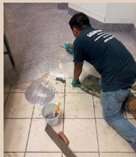
Applying a troweled system.
