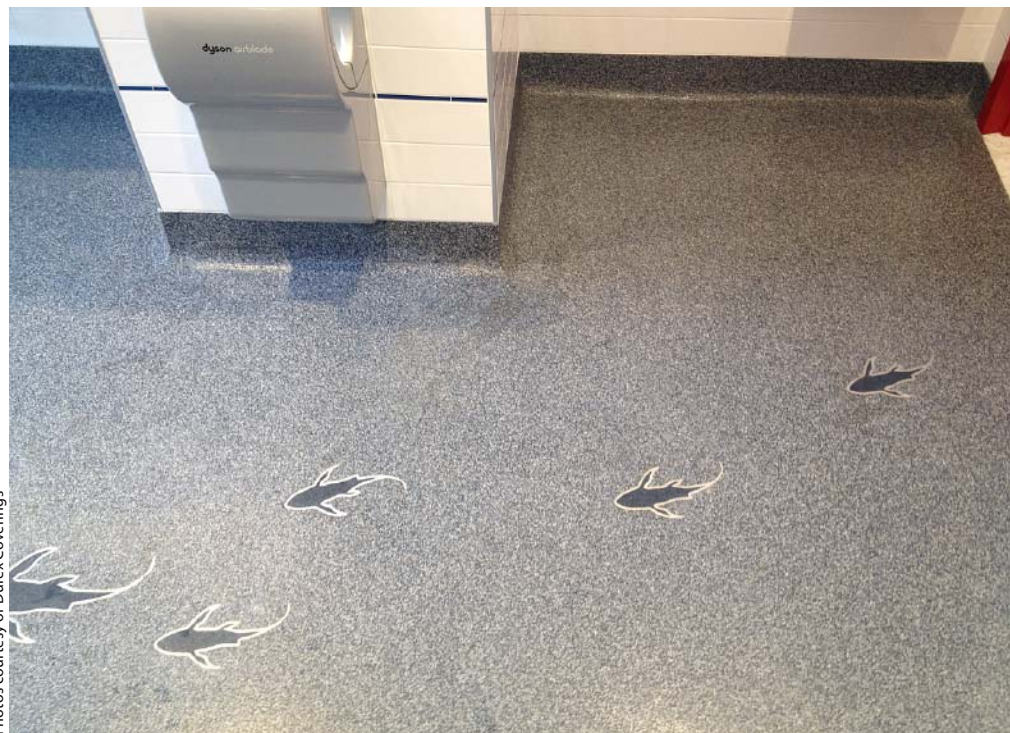
A trowelable epoxy mortar floor will have a speckled look, says Durex Coverings president Kevin DeCarlo.
