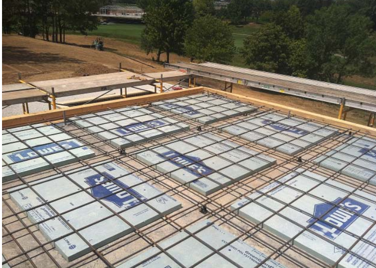
Polystyrene foam blocks, placed in forms to create a lightweight beamed deck.
