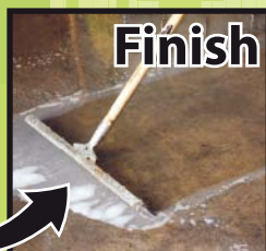
Urethane sealer on concrete floor
