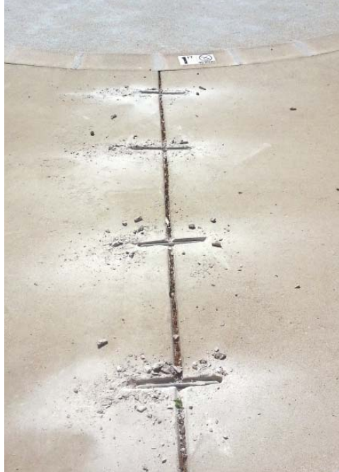
Concrete Product Resource staples are about a foot long and 5/8 inch in diameter.
