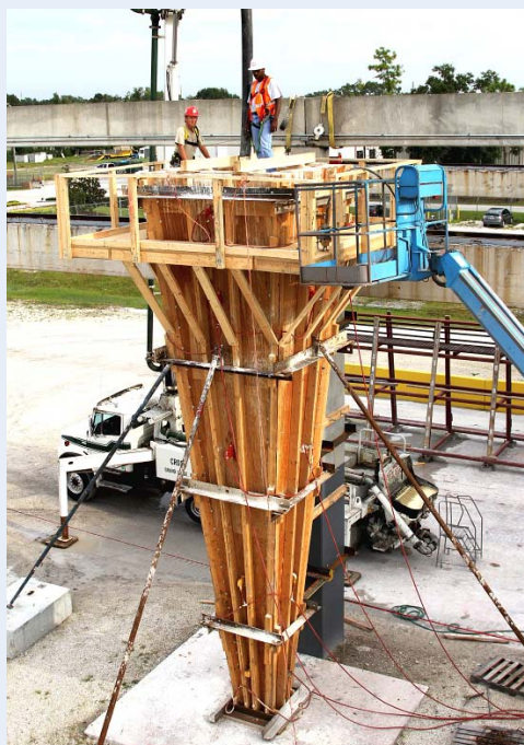
A pump was used to place concrete in formwork for the steeple for an LDS church in Davie, Florida.
