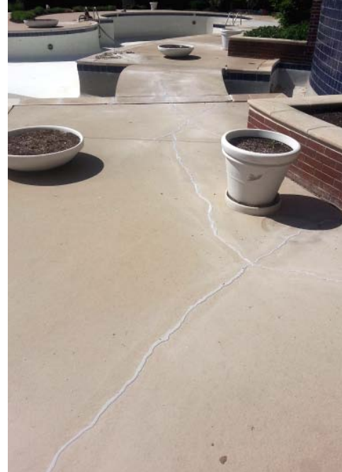
Cracks were chased and filled with epoxy before the microtopping was applied.
