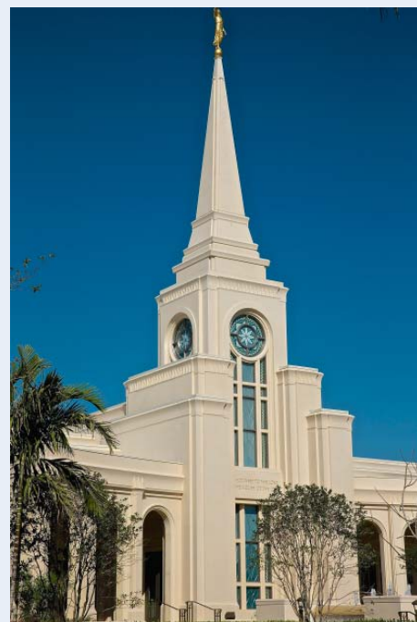
A void inside the steeple was created using a steel form to minimize the finished weight.
