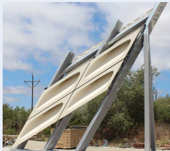
The completed panels and their steel frames are supported by a complex grid of structural steel members.
