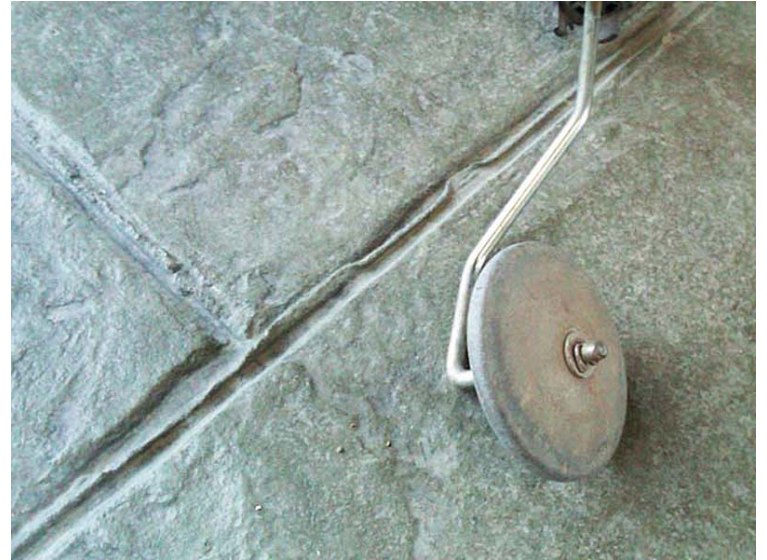
These sharp little fins appear between the stamps when stamping is done too early or the edges are tamped too hard.
