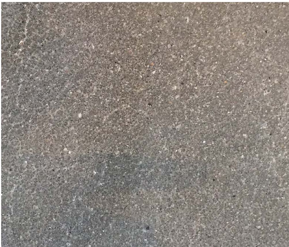
Seen here is a salt-and-pepper reveal with no small aggregate. There must be small to medium aggregate exposure or it is a CPAA Aggregate Exposure Class B- Fine/Sand Aggregate Finish.
