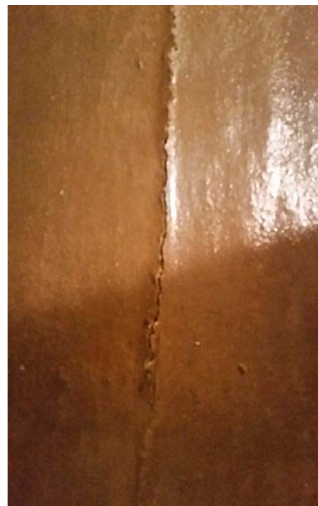
Inadequate preparation can cause cracks along the wooden subfloor seams to migrate through an overlay.
