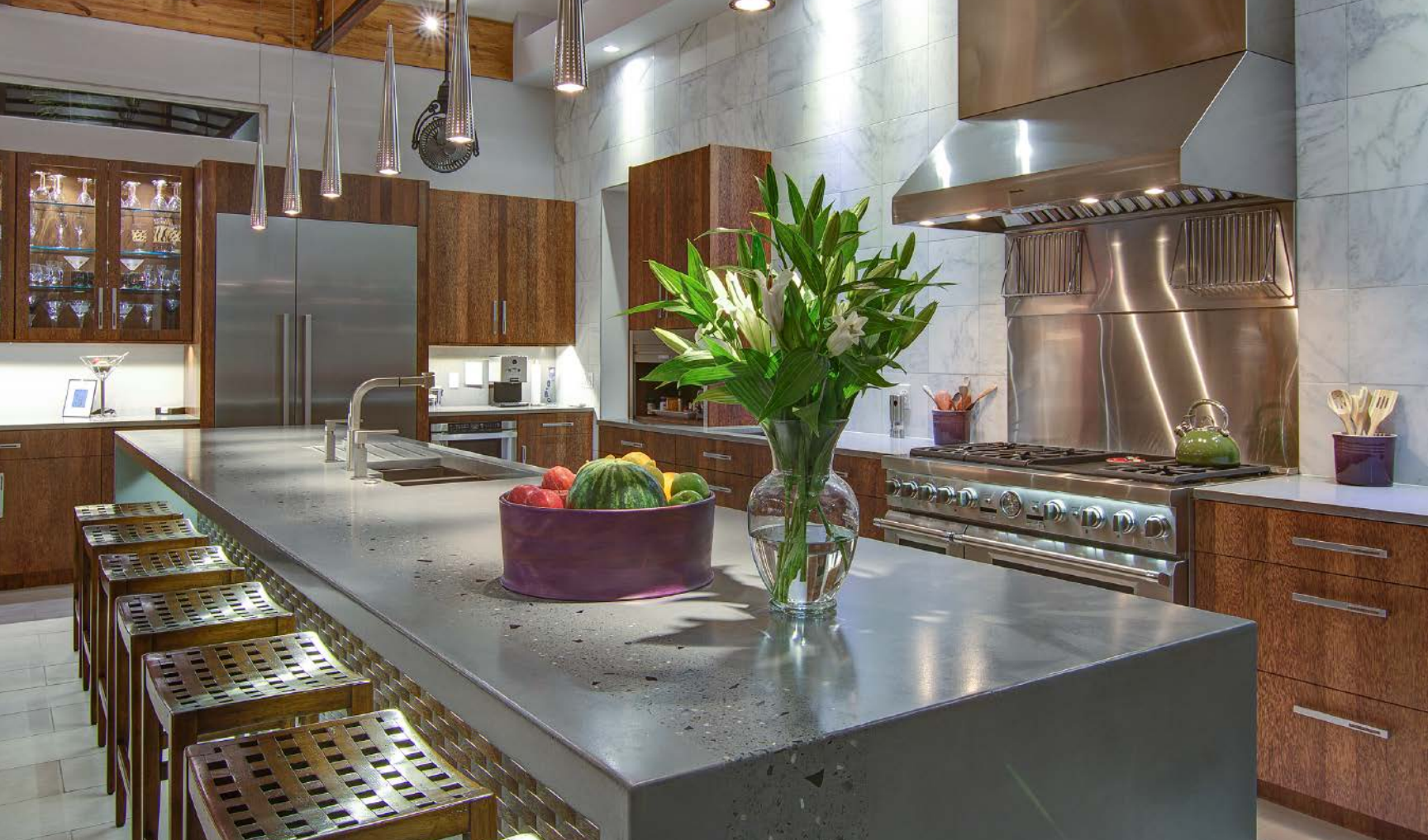
Here's an example of a seamless, precast GFRC island with waterfall ends.
