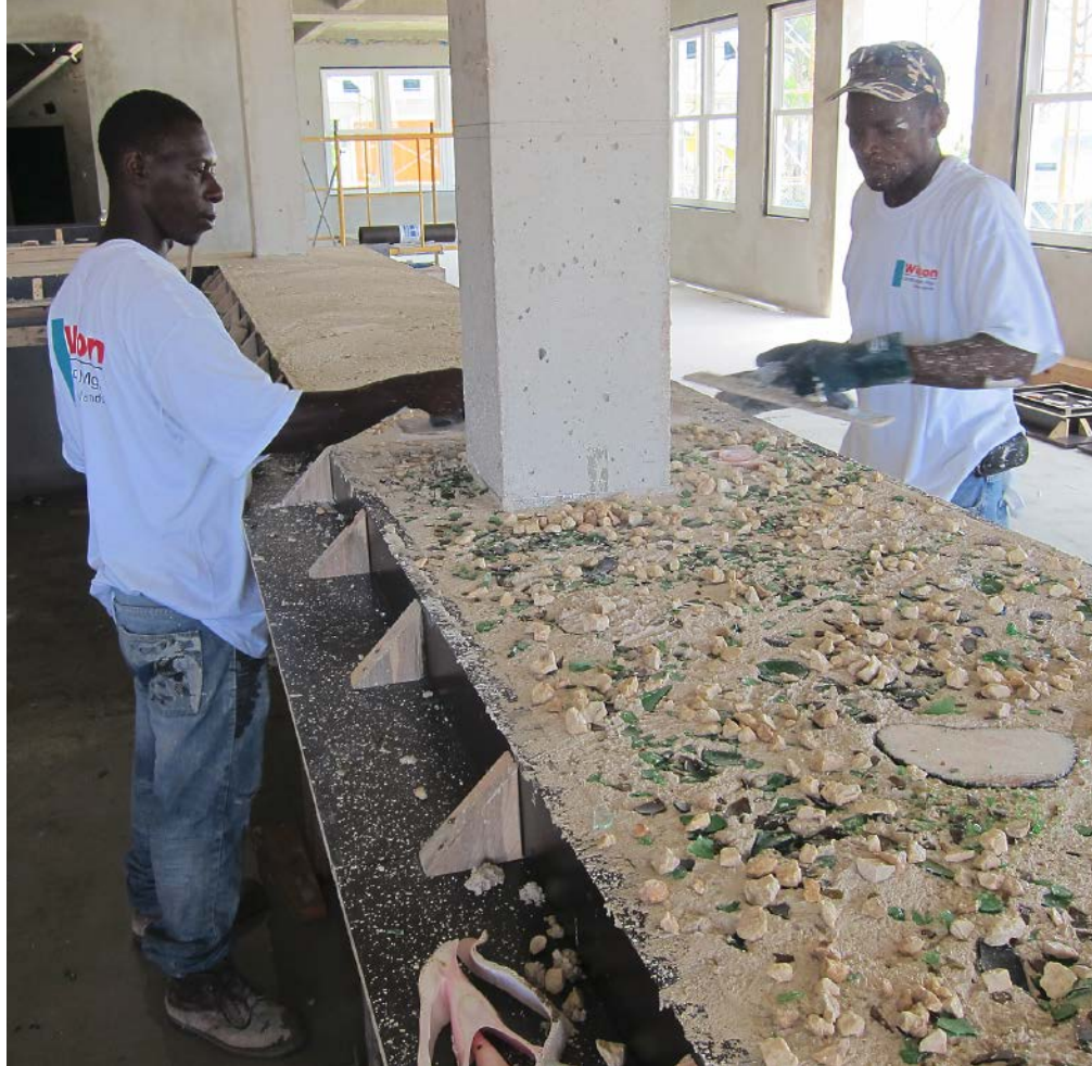
Workers seed and float in a large amount of decorative aggregate.
