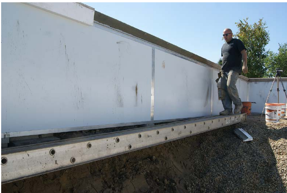
Prebuilt scaffolding inside the pool allows for easy access to the deep end while working.
