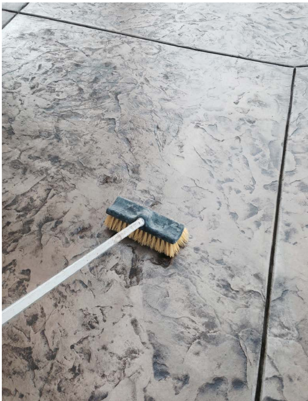
After applying a coat of new sealer over an existing coat, use a chemical-resistant broom to agitate the surface. The agitation will not only reactivate the old sealer but it will also mix the old with the new.
