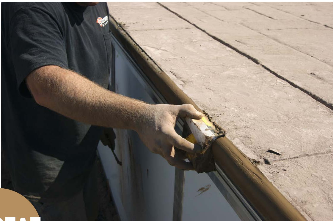
Jason Geiser applies color hardener slurry to a coping face.
