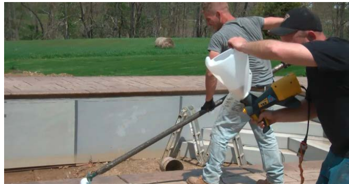
Jason Geiser applies traction additive using the broadcast gun while the second coat of sealer is still wet. Jason Hershberger immediately back-rolls it.
