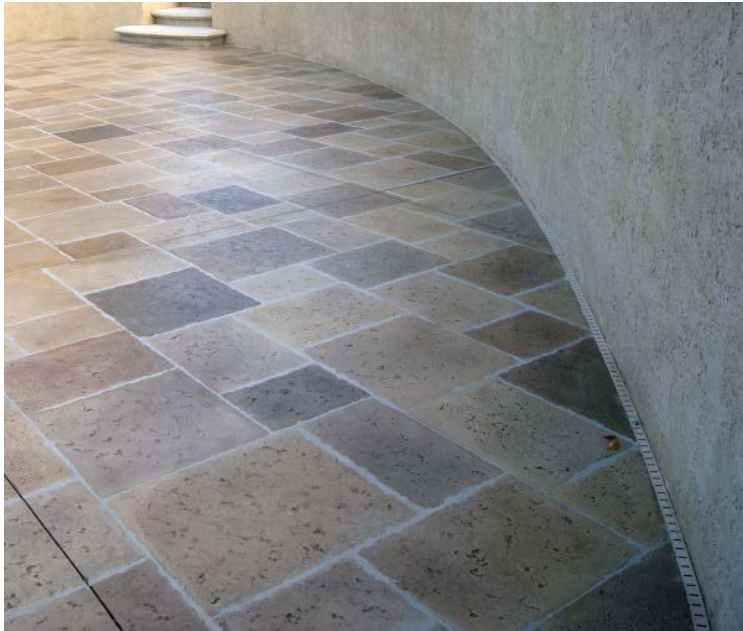
Deck drains such as the one around this wall allow the decorative concrete professional to be creative with design, yet still provide an outlet for water.
