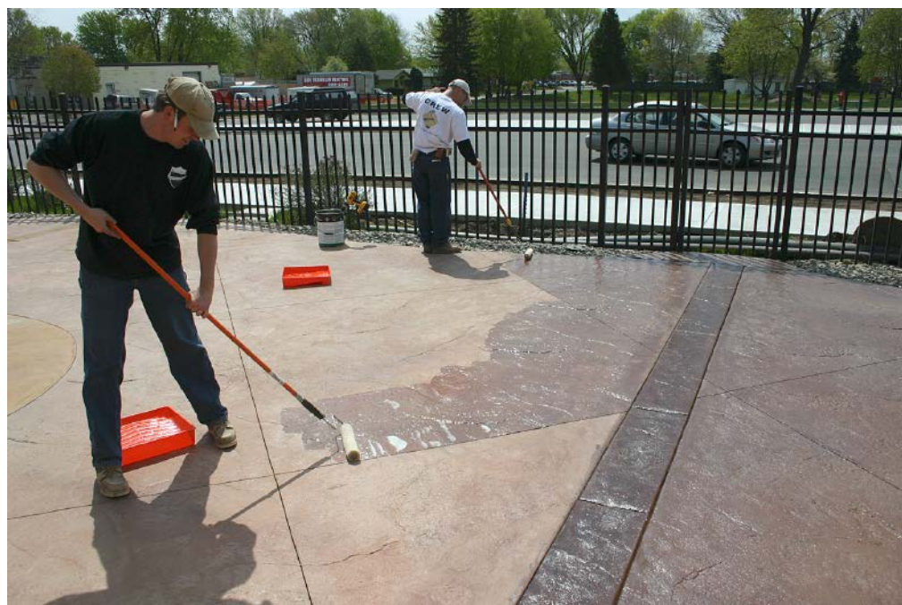
Crew members apply and back-roll a solvent-based acrylic sealer during the open-time phase.
