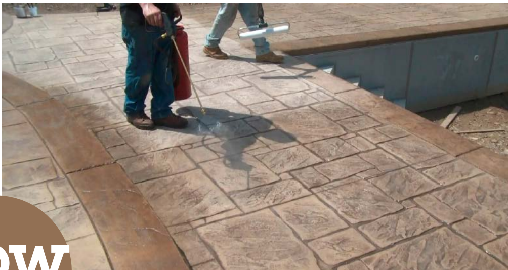
The author recommends D-One Plus sealer for saltwater pool decks. Here, the first coat of sealer is being sprayed on and back-rolled.
