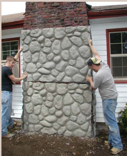
CMJ can cast lightweight sheets of veneer stone in a host of sizes and finishes, including fieldstone (left) and stack stone.
