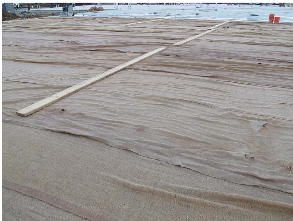
Burlap works great as a wet curing agent as long as it is evenly placed with very little overlap. This process keeps the slab’s surface cool and moist, allowing for an even and dense cure.
