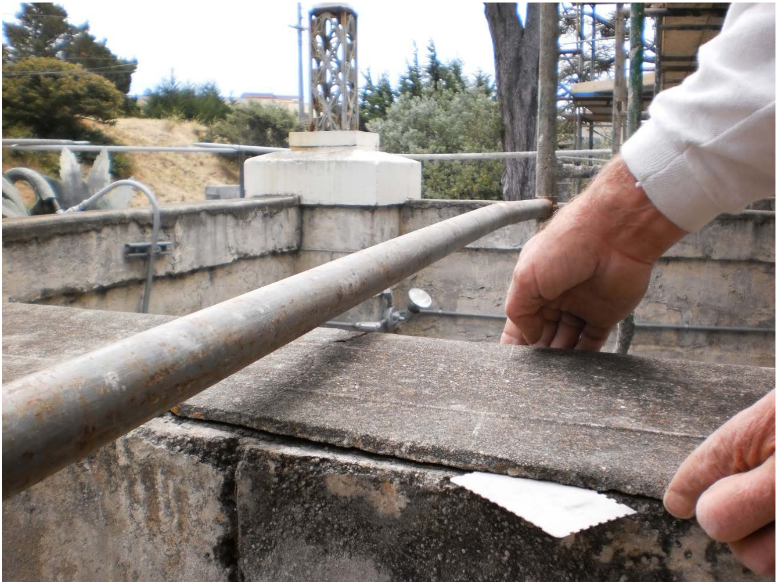
Replacing damaged or missing parapet caps, which prevent water from infiltrating wall systems by shedding water off the building.
