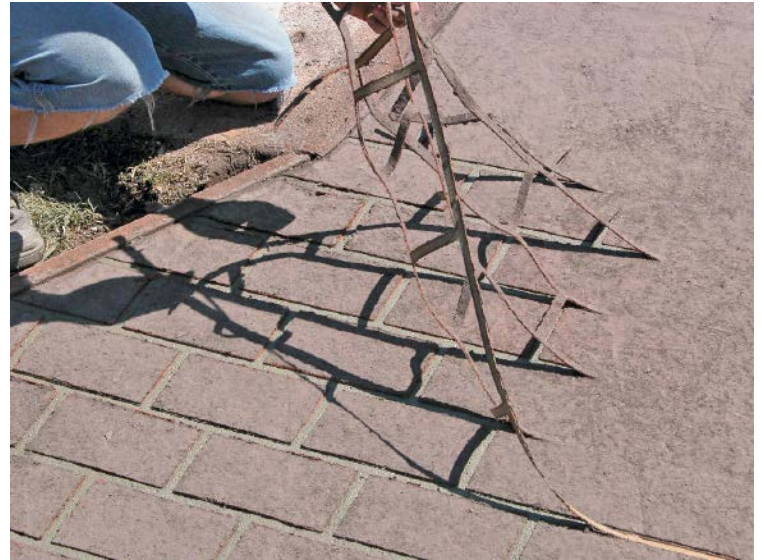
It's imperative to remove the stencil immediately after texturing.
