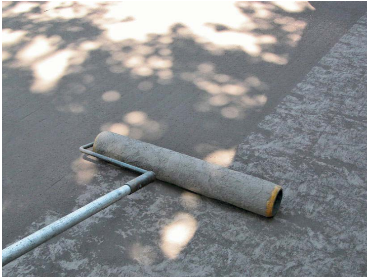
Texture is applied with a roller over powdered release. Although you can barely see it, a stencil is in place.
