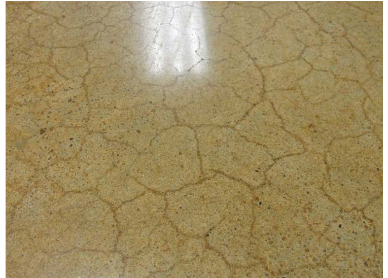
When rapid curing occurs, a concrete slab usually exhibits "craze" or "map cracking." This type of cracking can also occur on hot windy days when the surface cures before the contractor can apply any type of cure.
