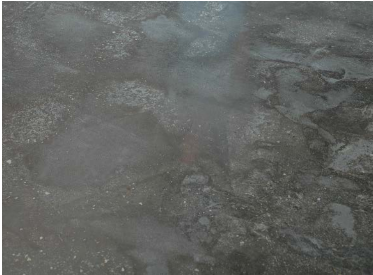
Curing with Visqueen creates a unique pattern on the concrete because the areas where the plastic touches retain more moisture and are darker than those that aren't in direct contact with the plastic. The only remedy to this look is to grind for exposed aggregate.
