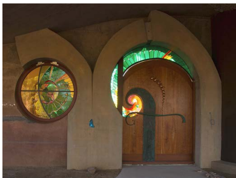
Type K shrinkage-compensating concrete enables accurate forming of irregular window openings, such as these.
