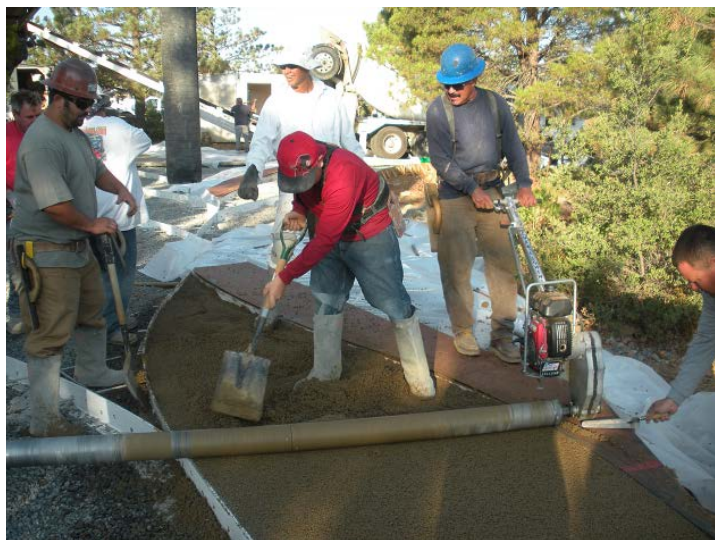
The crew pours a section of the pervious driveway, compacting it with an aluminum roller screed.
