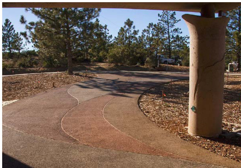
The pervious driveway is colored with five different colors to match parts of the house.
