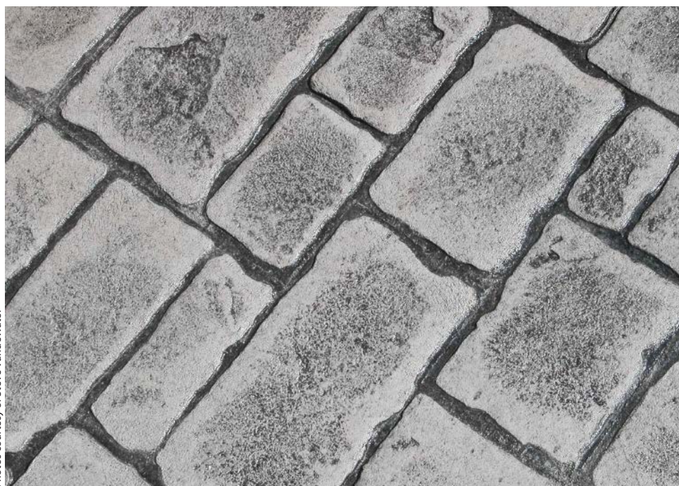
On this poorly textured surface, there is no texture near the stamped joints.
