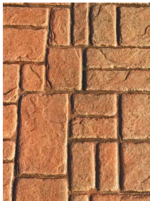
Here is an example of proper imprinting, where the stamped texture goes all the way to the stamped joints.
