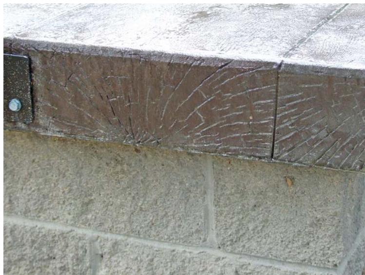
The platform edges were stamped to mimic the grain of aged timbers.
