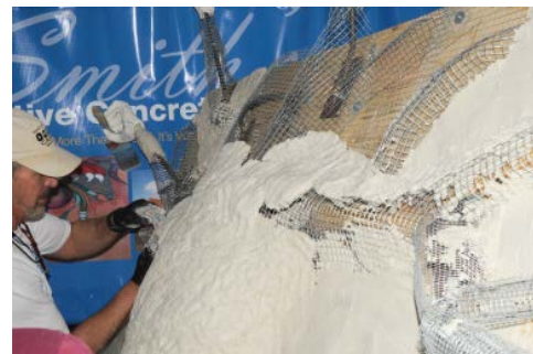
For high-relief areas such as the trunk and limbs, thick pancake-like slabs of Smith's 4-n-1 Overlay are padded out and pressed onto the mesh.
