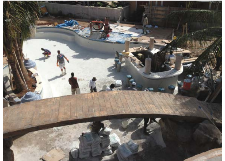
The bridge was formed with a plywood form, 2-by-4s and wood poles for support. A double layer of 5/8-inch rebar and 8 inches of concrete were specified.
