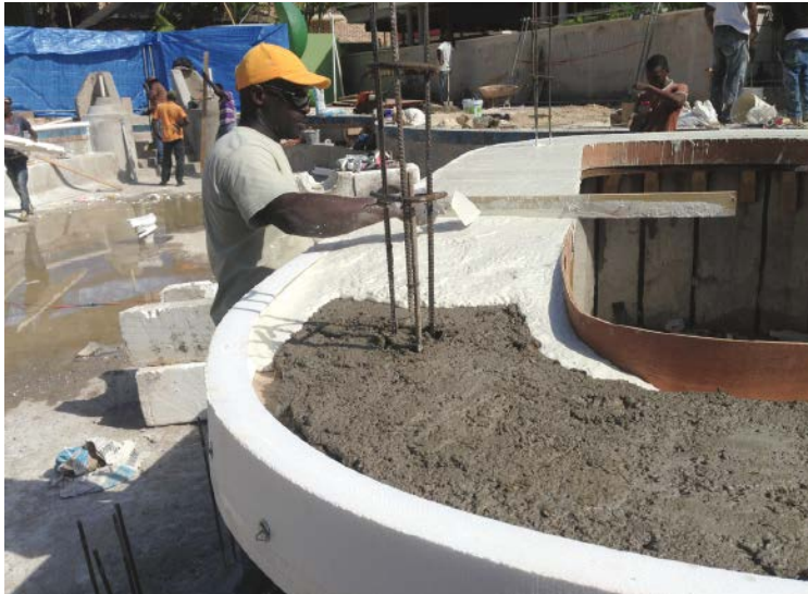
Stegmeier forms provided a bullnose finish on the pool coping and bar top. A steel-reinforced concrete core was capped with a white cement mortar mixture.
