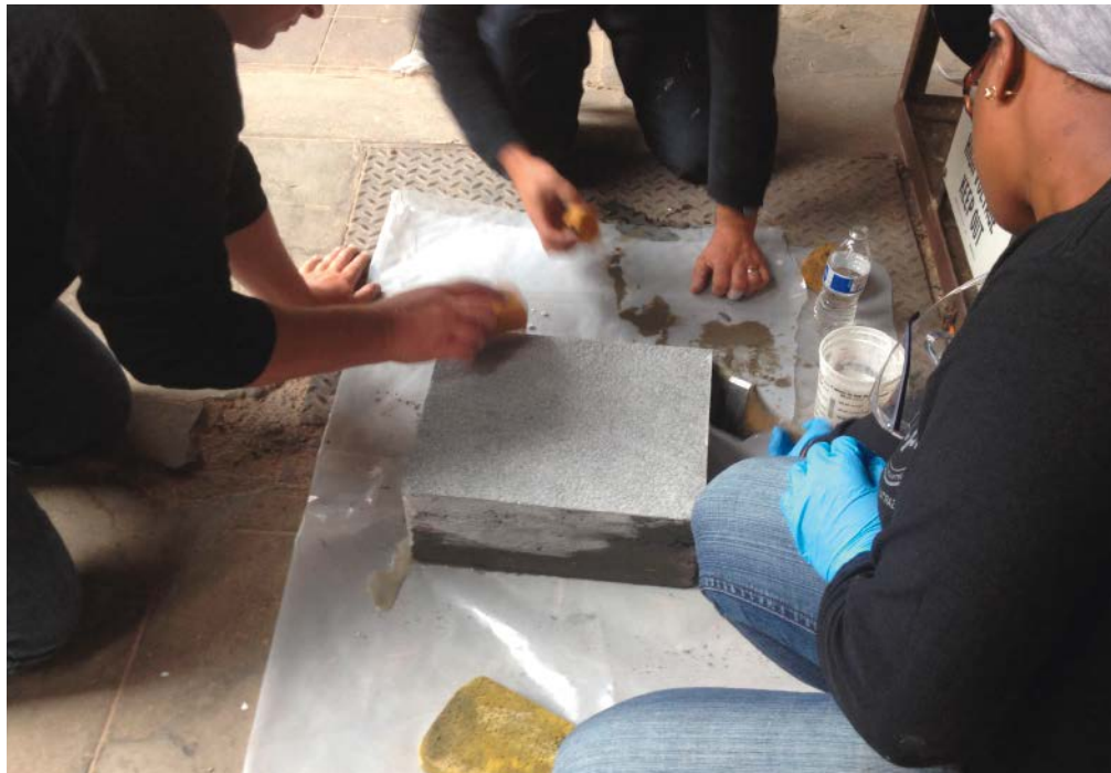
Students color a sample that was cast using the texture skin they helped to make. The samples will be used when they pour footings for the wall panels.
