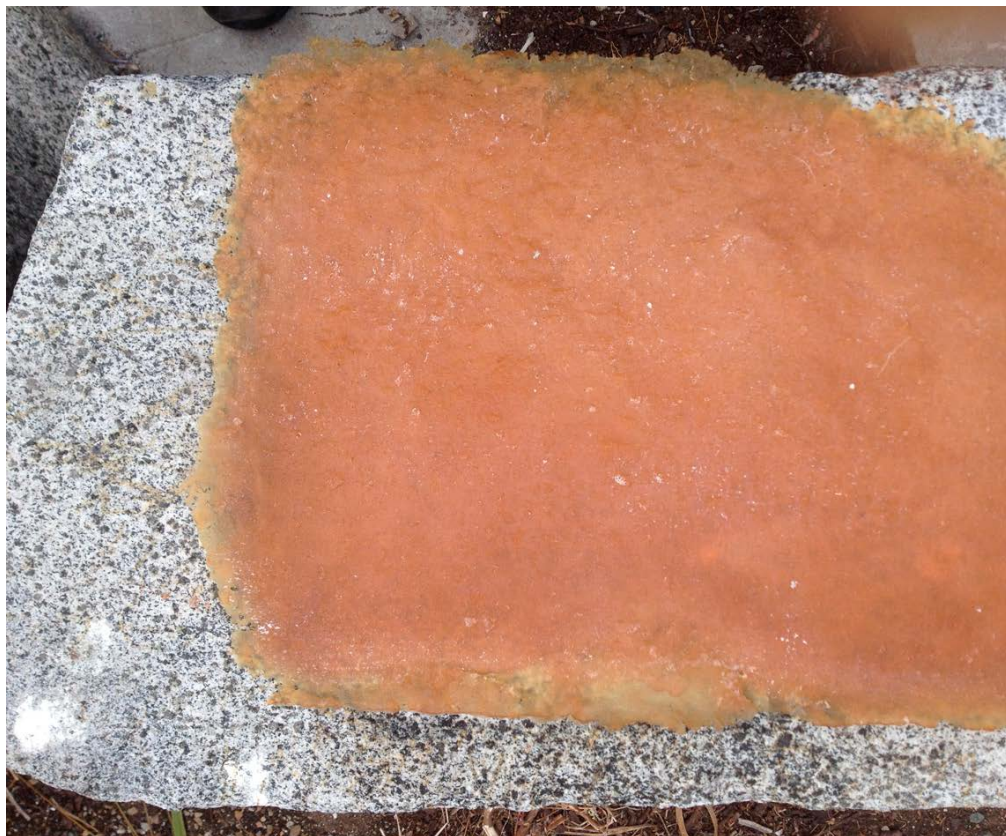
A de-molded texturing tool rests on a piece of textured concrete.
