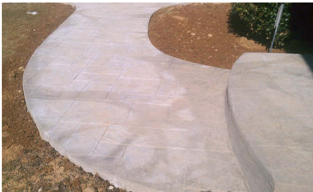
Curing blankets placed with air gaps leave blotchy marks on the stamped concrete walkway.
