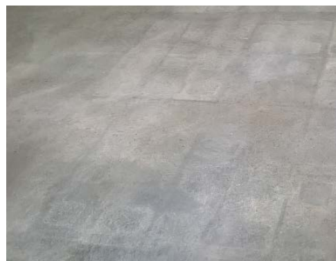
Concrete blocks placed on concrete a few days old create a curing differential resulting in the permanent outline of the blocks in the floor.
