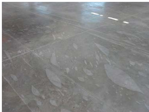
Plastic curing sheets with wrinkles create the classic "leopard spot" pattern in this gray concrete floor.
