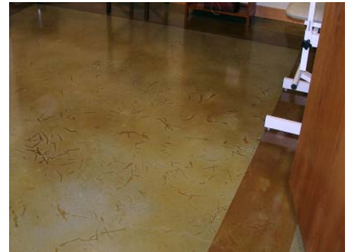
Alfalfa soaked in brown acid stain, drained and scattered across a lighter color.
