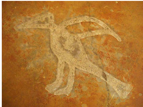
Acid etching of stain through cut felt fabric.
