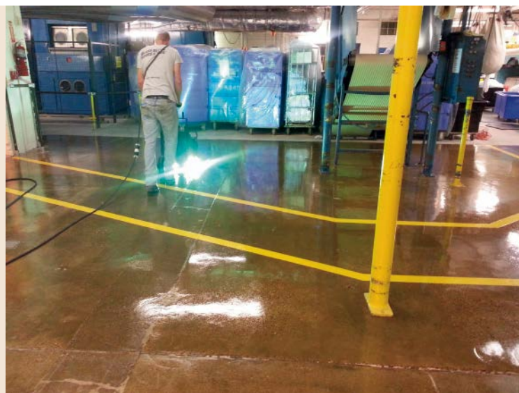
Although it looks highly polished, the floor in this laundry facility was taken up to a 100-grit finish and coated with a UV-cured coating.
