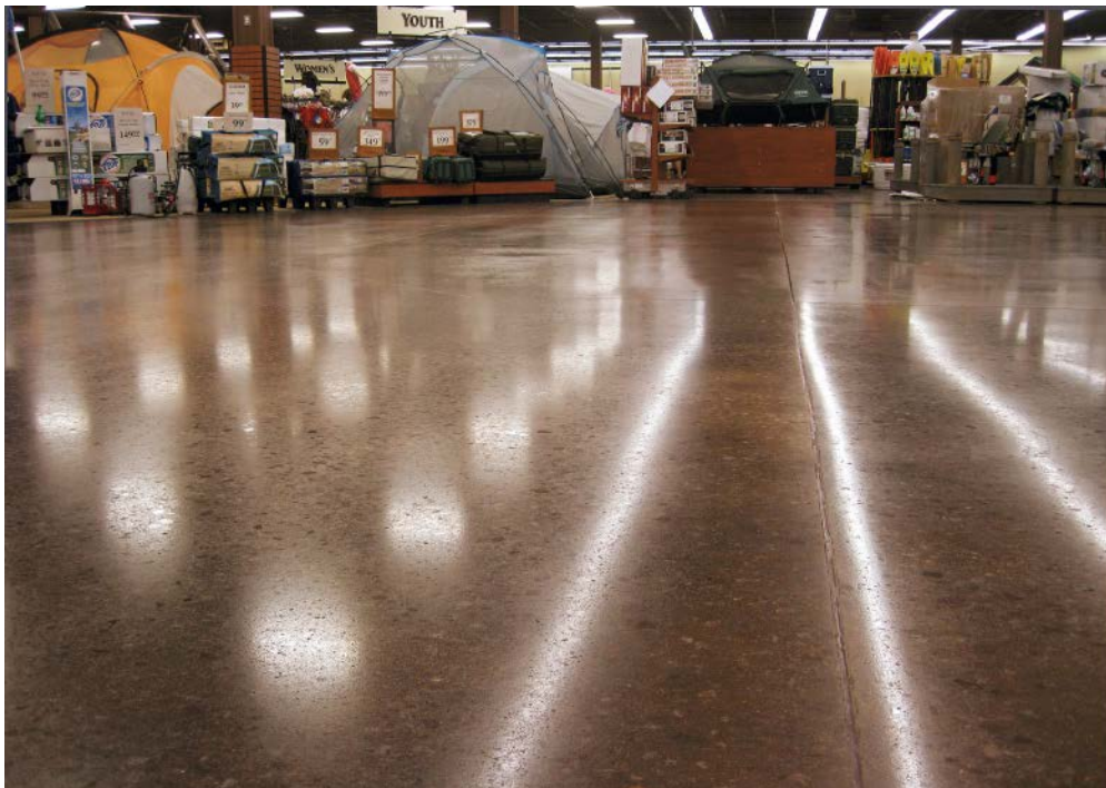
A proprietary acrylic copolymer modified with a silicate hardener was applied as a sealer, or “guard,” on this polished concrete floor.
