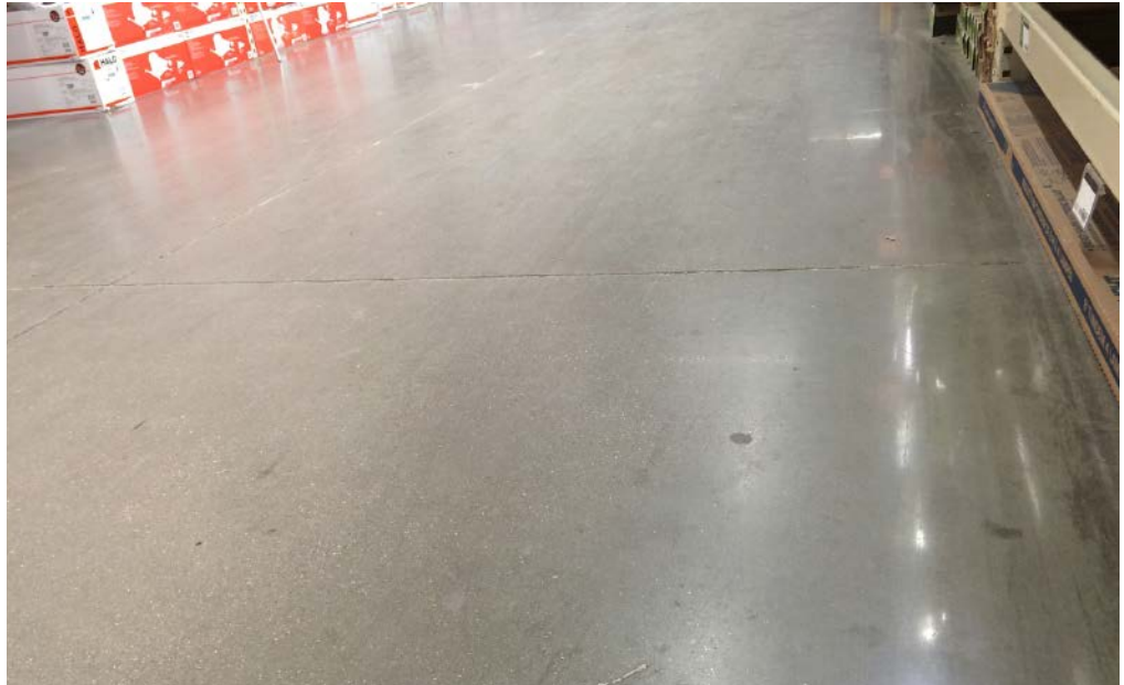
Foot traffic patterns in the middle of this aisle show where the semi-topical sealer has worn off in a short time.
