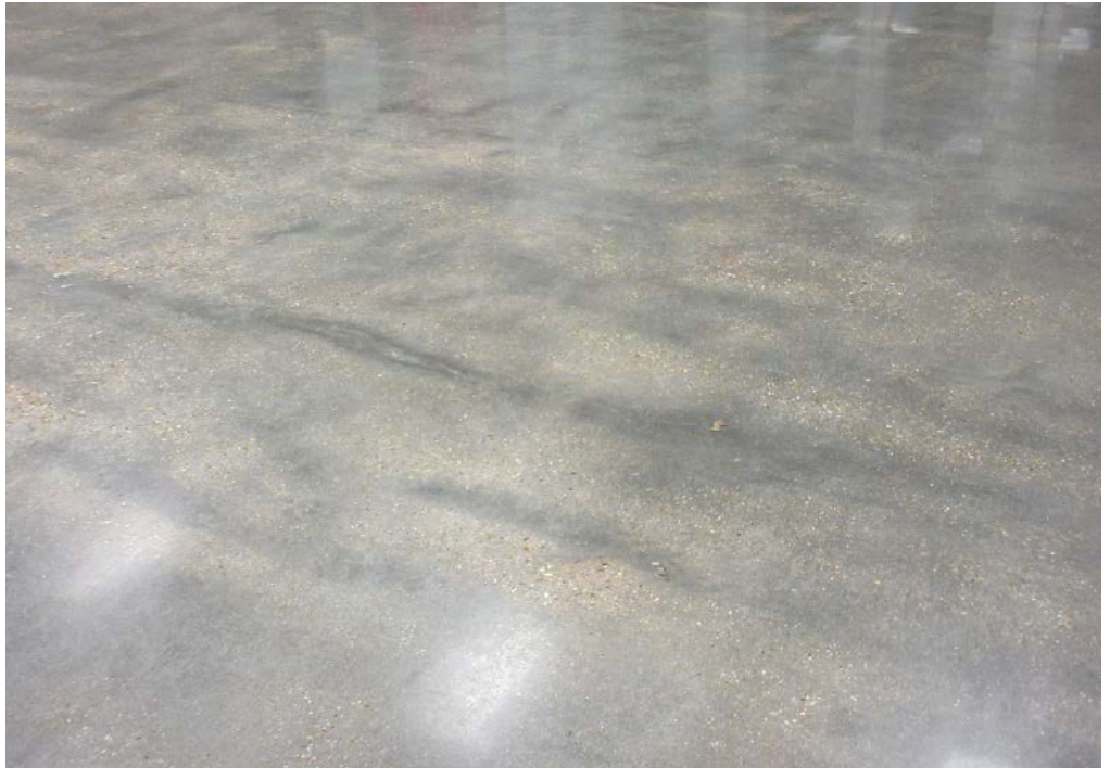
Low FF numbers, as was the case in this remodel, generally result in many random high and low spots highlighted by the concrete polishing process.
