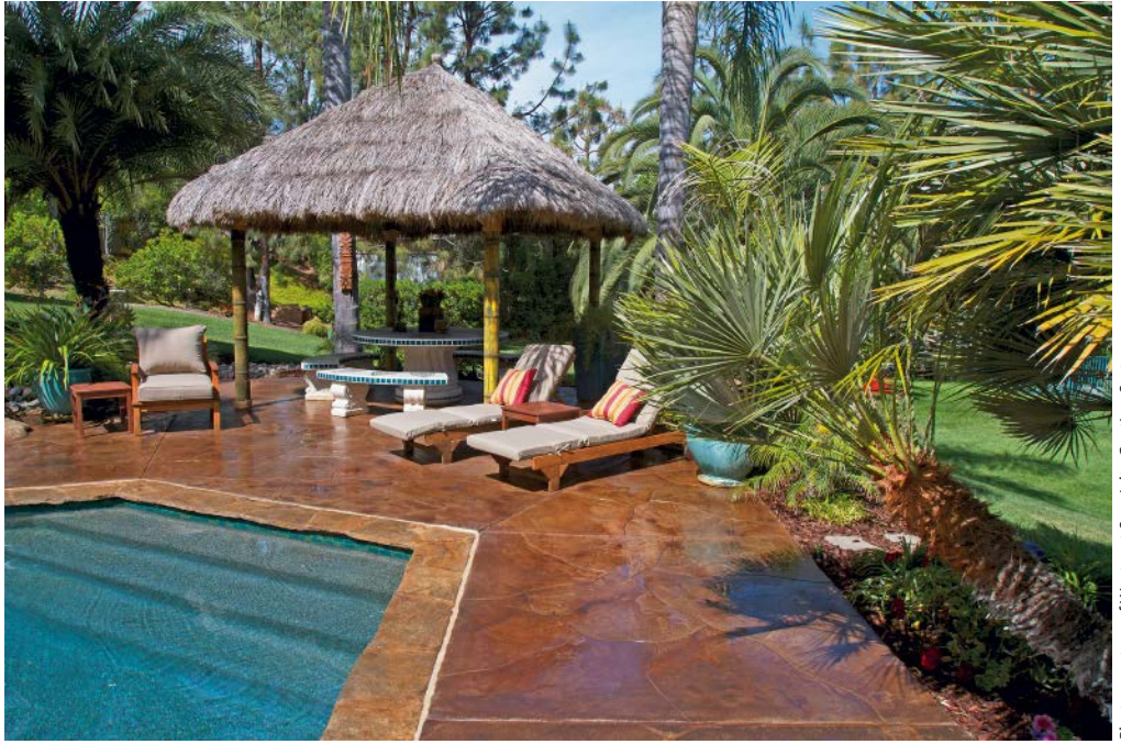
A polymer-modified cementitious coating with acrylic topcoat is a viable option for resurfacing and enhancing existing concrete. This type of coating system can produce a smooth or textured finish, and simulate tile, flagstone, slate and other surfaces.
