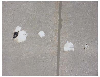
Existing underlayments must be removed and holes repaired with a material that will hold up to traffic.
