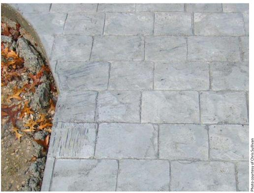
Any dragging or sideways movement of tools can lead to the colored release powder streaking.
