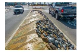
Surrounding the roundabout, 12 islands of various shapes and sizes are fashioned out of a proprietary concrete mix. Each is acid stained in multiple colors and contains starfish, shells, small pebbles and a mix of large flat rock. Acid-stained veins on most of these steep-graded surfaces make them look like vertical concrete, Ralston notes. "To make veins that would not run down in errant patterns everywhere, we had to develop a staining system."
