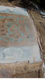
but for the very center of the building approximately midstream — we changed the mix and started pouring a 3/8 inch, 5.5 sack pea-gravel mix" to create a washed aggregate look for the streambed.
