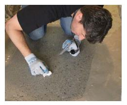
The **RetroPlate Concrete Polishing System** (www.retroplatesystem.com) was among the first in the industry to combine diamond grinding and polishing with a one-application densifying sealer that proponents say never needs to be reapplied. The patented process permanently strengthens concrete floors while making them highly reflective and resistant to abrasion and impacts. RetroPlate can be used on new or existing floors in residential, commercial and industrial settings.
