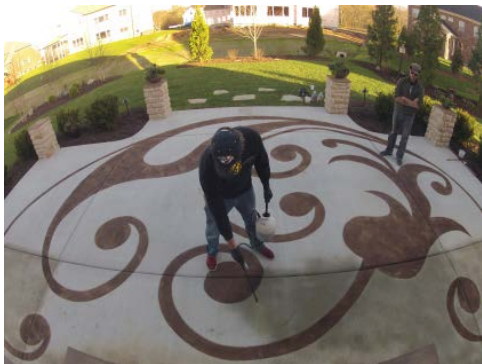
Rick Lobdell draws, saw cuts and stains the design on this patio in Brentwood, Tennessee. The design was based on a pattern found on an area rug elsewhere in the home.
