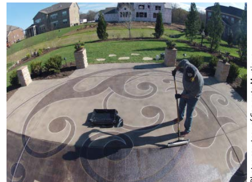
Rick Lobdell draws, saw cuts and stains the design on this patio in Brentwood, Tennessee. The design was based on a pattern found on an area rug elsewhere in the home.
