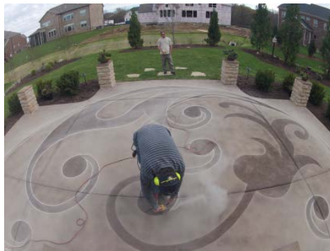
Rick Lobdell draws, saw cuts and stains the design on this patio in Brentwood, Tennessee. The design was based on a pattern found on an area rug elsewhere in the home.
