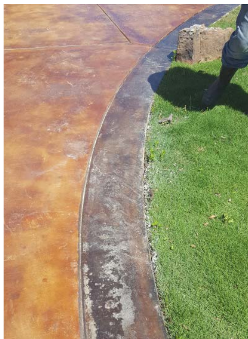
The lawn surrounding the driveway was saturated, leading to moisture issues under the acid-stained driveway.
