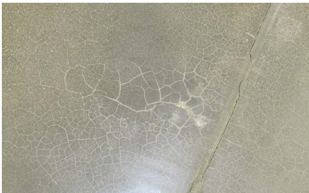
This is what delamination looks like before it's repaired.
