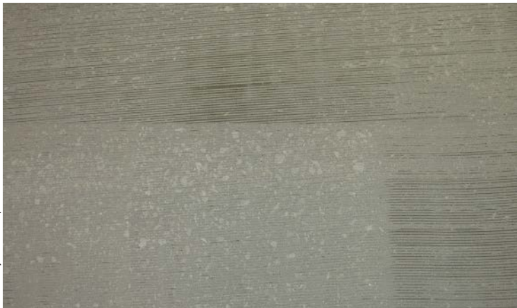
Here's a profile of a delaminated area after the shaver removal.
