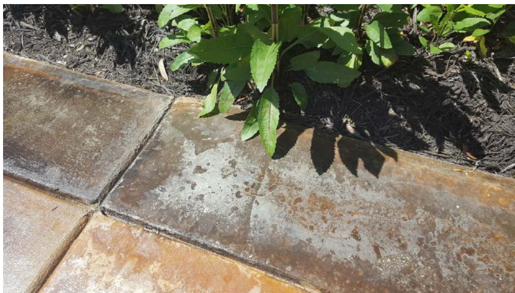
Moisture from irrigation in the raised planter beds next to the driveway created both surface and subsurface hazing and whitening on the acid-stained driveway.
