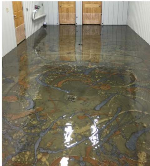
The second coat of PT1 epoxy with the metallic additives is applied.
