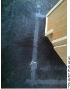
Blue painter's tape used to mark off the location of cabinetry on an integrally colored concrete floor leaves glue residue when the tape is removed. Ghosting occurred after the sealer was applied.
