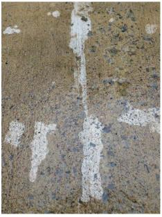
Car tire cleaner that spilled on a driveway is not evident until a sealer is applied.
